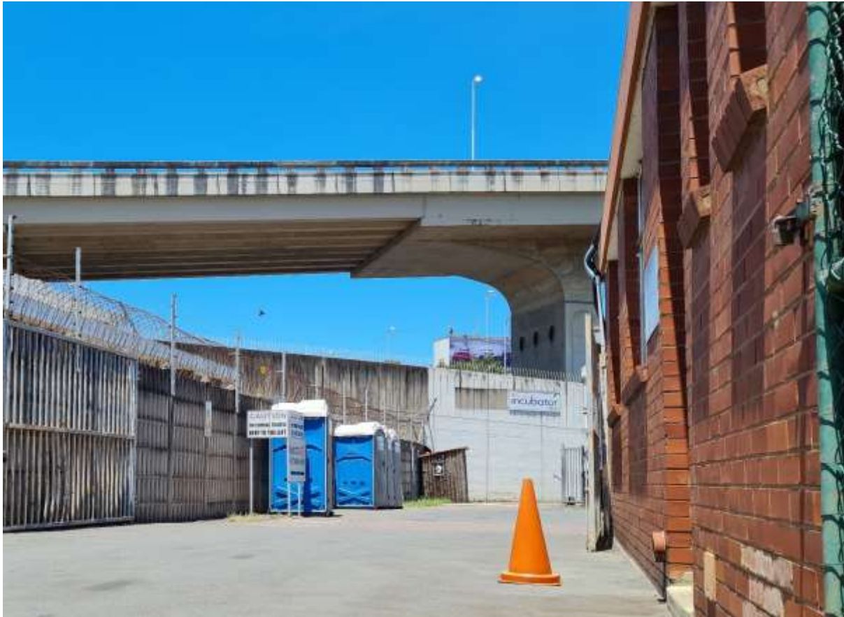
Figure 1 David Webster Street Hangs Over the Asiye eTafuleni Offices in Warwick.
