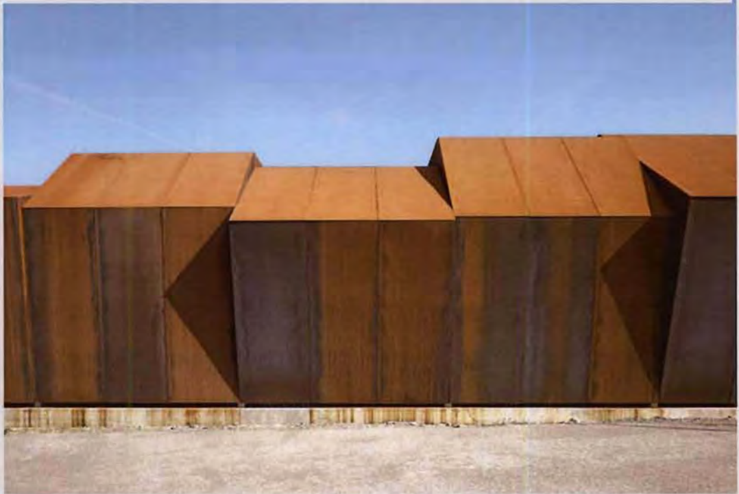
Corten Steel Elevation of the Utilities Building: 33kV Primary Substation Travis Street, Manchester (Source: www.archello.com )
