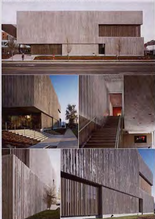
Clyfford Still Museum: Images of Facades and Internal (Source: www.alliedworks.com )
