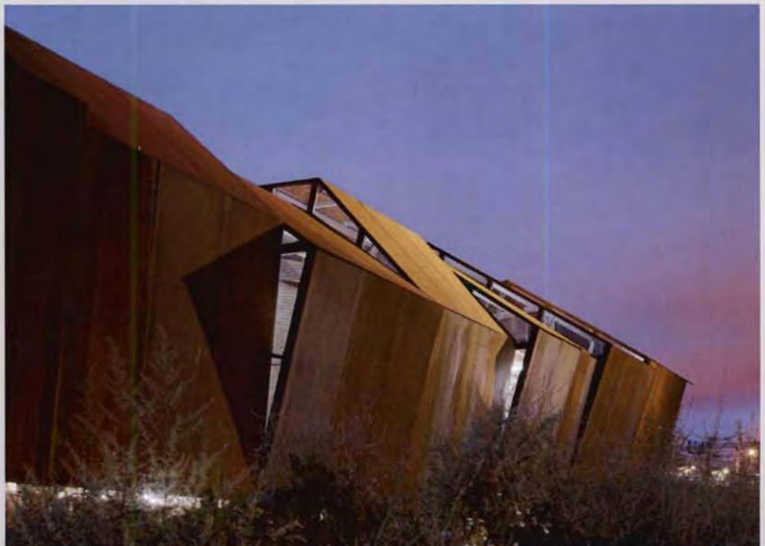
Side of the Utilities Building: 33kV Primary Substation Travis Street, Manchester (Source: www.archello.com )
