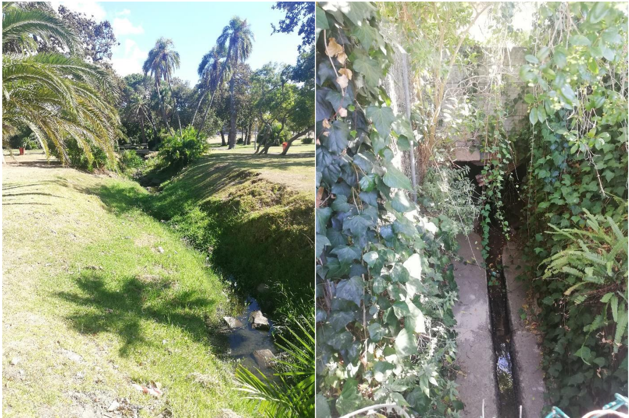
Figure 6-2: Examples of Irregular (left) and Constructed Channels with Regular Sections (right)
