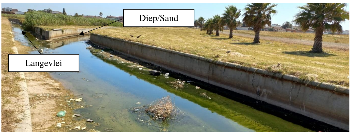
Figure 7-8: CR21 Sampling Point (after confluent of Sand River and Langevlei Canal)
