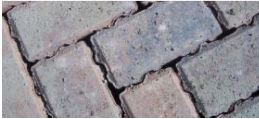
Figure A-4: Permeable Pavement showing gaps between pavers (CHI, 2019)
