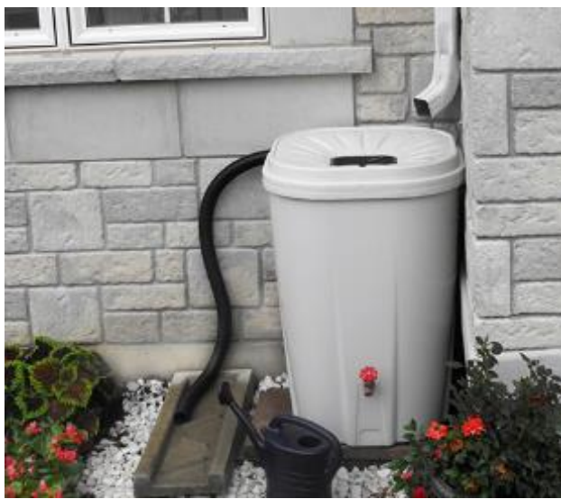
Figure A-3: Simple Rainwater Harvesting System (Left). Rainwater Harvesting Conceptual Model (Right) (CHI, 2019)
