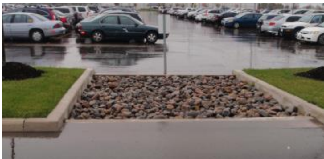
Figure 2-8: Infiltration Trench (CHI, 2019)
