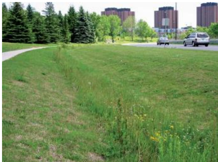
Figure 2-6: Vegetated Swale (CHI, 2019)
