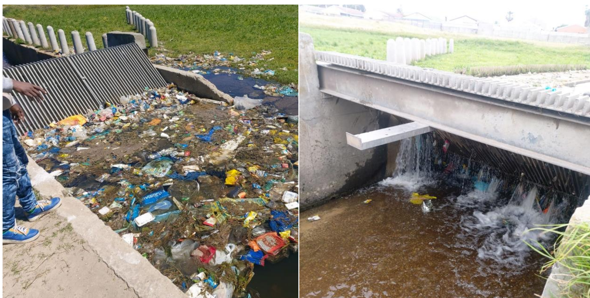
Figure 8-19: Upstream (left) and Downstream (right) of Sand River Litter Trap
