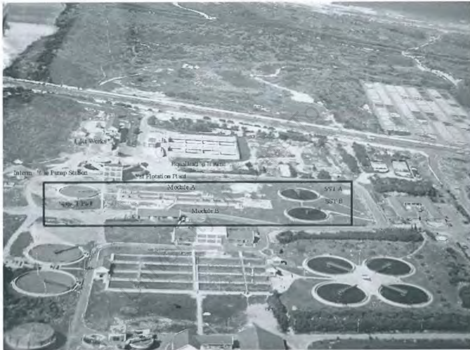
Figure 3.1 : Stage 1 plants in relation to the rest of the Mitchell's Plain WWTP.
