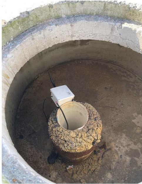
Figure 3-23: Installed Water level Sensor in the 45 m deep Borehole
