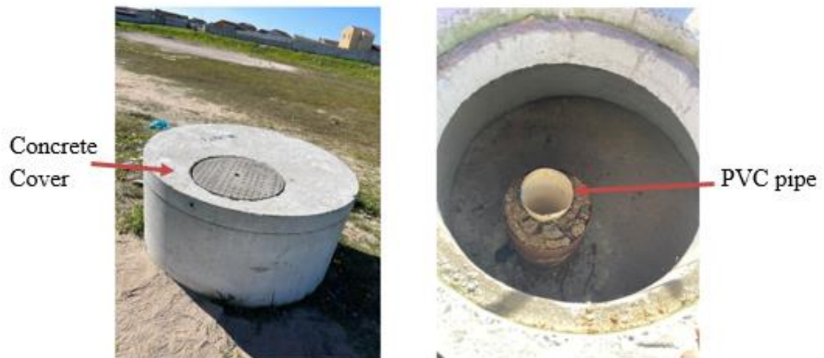
Figure 3-16: CCT MON71 Borehole
