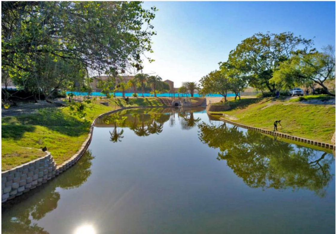
Figure 2-18: On-site Retention pond located at CPUT Campus
