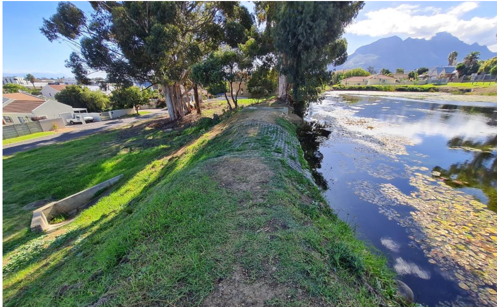
Figure 45: A retention pond showing an outlet
