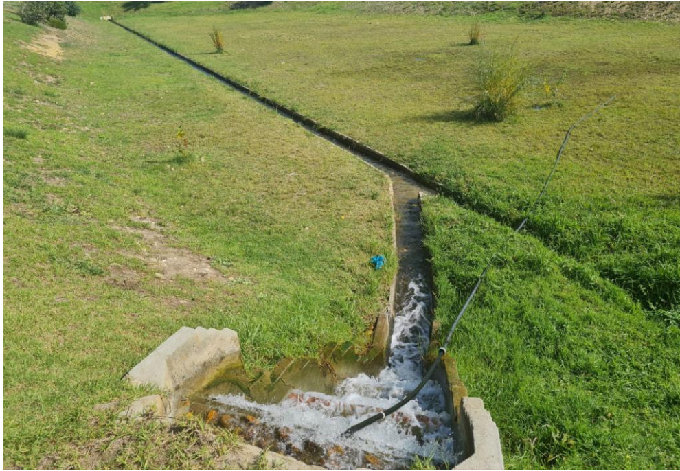
Figure 47: A vegetated detention pond showing the inlet and a concrete lined canal through the pond
