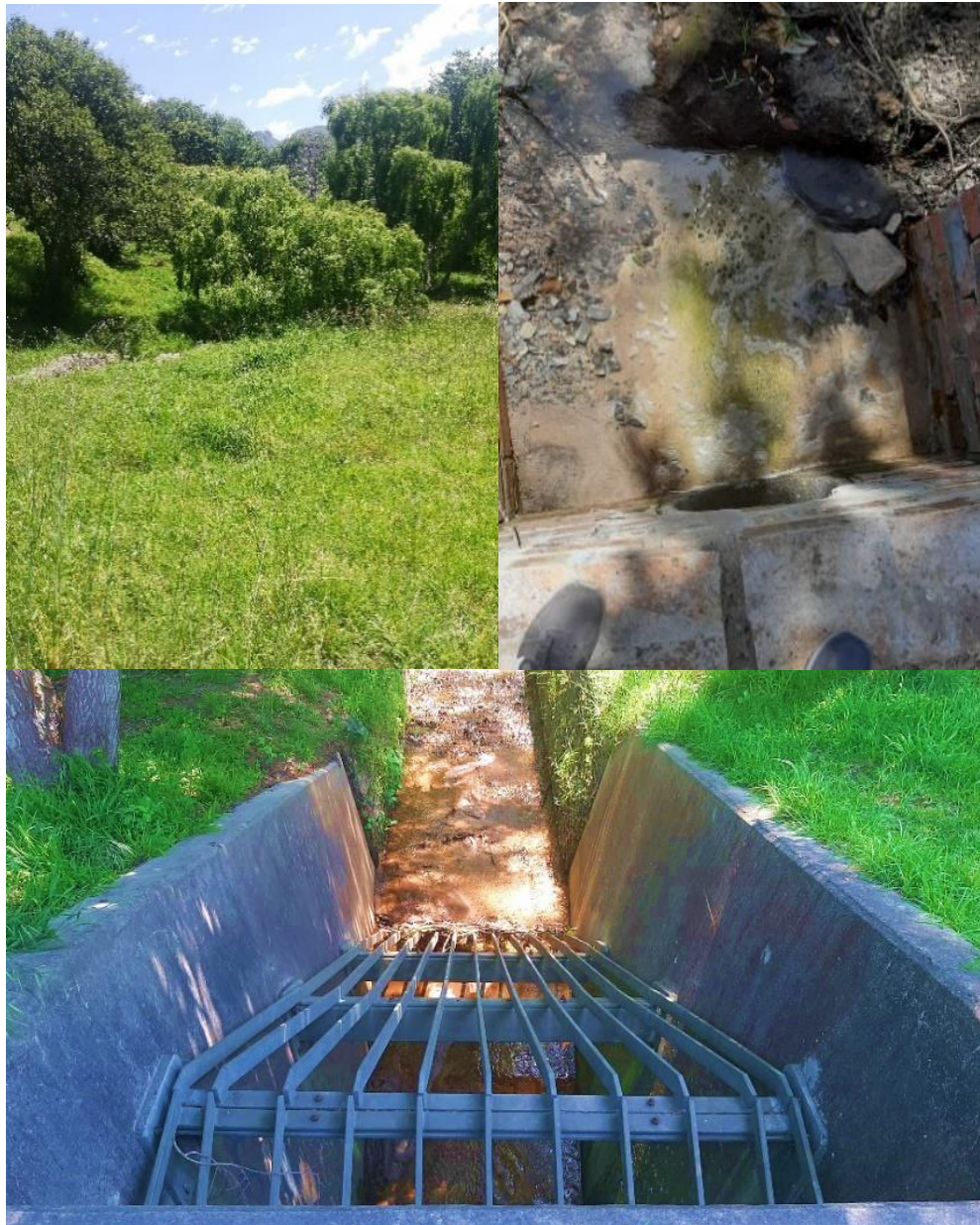
Figure 42: A vegetated detention pond along a greenbelt, with the inlet and outlet
