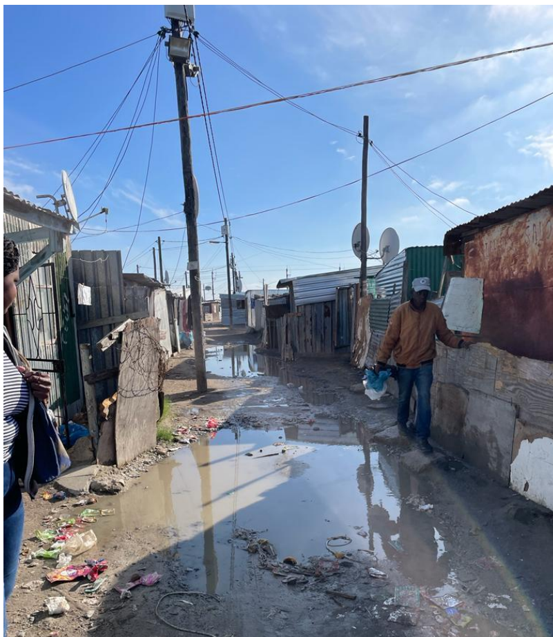
Figure 25: An example of an informal settlement with stormwater drainage challenges
