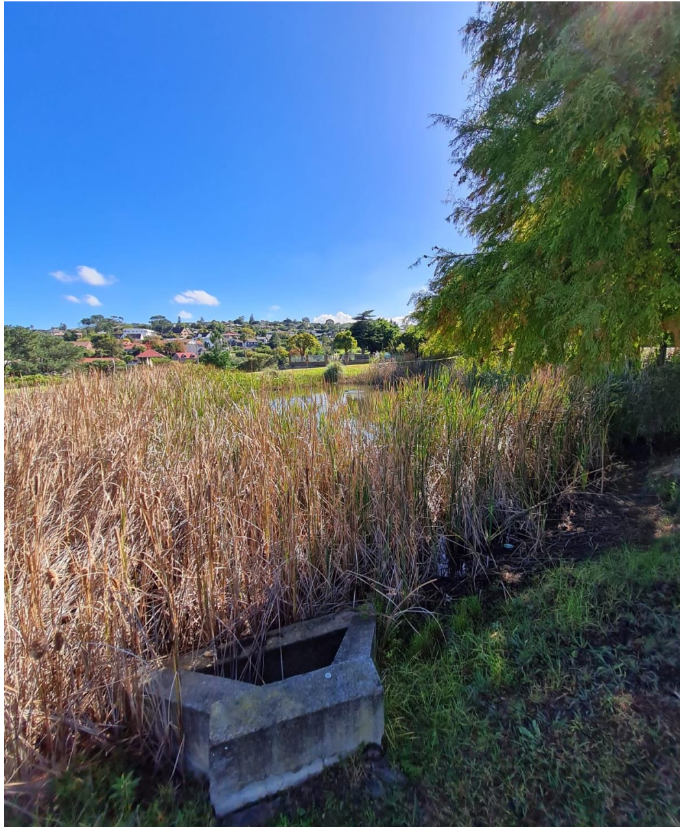
Figure 49: A retention pond next to a major road showing the outlet
