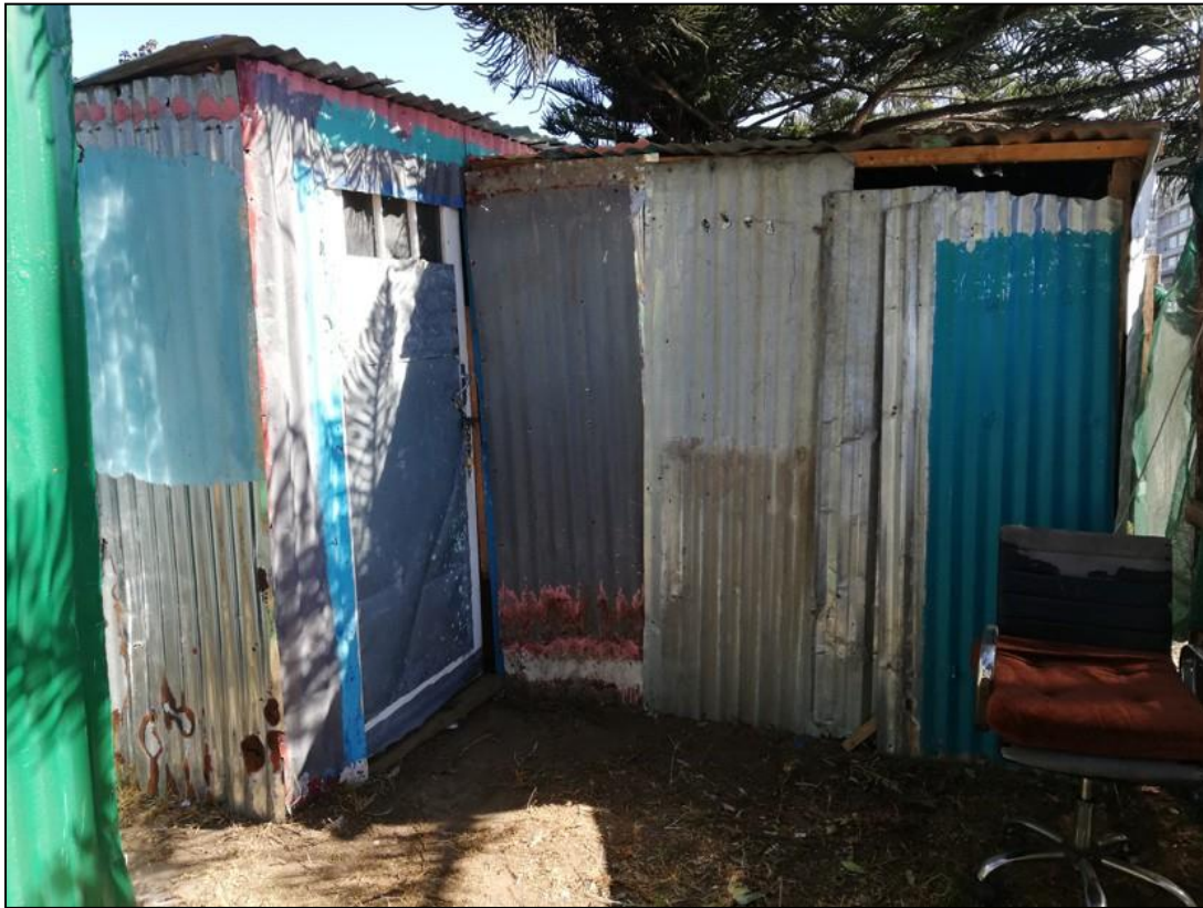
Figure 27 A metal sheet nailed across this glass-paned doorway prevented anyone from looking inside (source: Author, April 2021)
