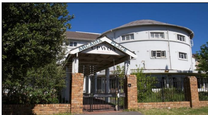
Figure 4 Arcadia Place old age home before its demolition (source: (Levy & Hendricks, 2019)
