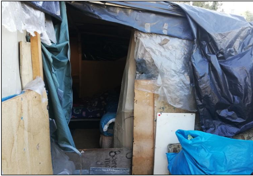
Figure 26 A rolled up doorway to the right of the entrance to this home could be pulled shut when needed (source: Author, April 2021)
