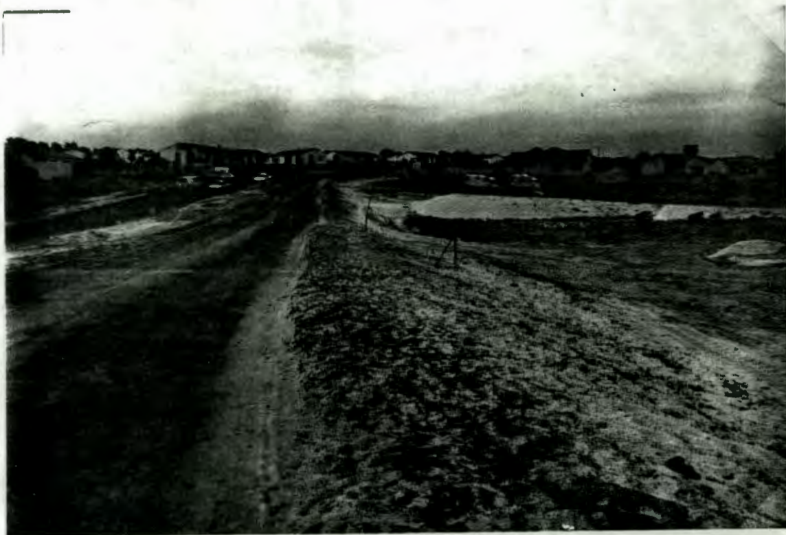
Plate 4: Road widening and construction (Kenridge), with builders' sand next to Elsieskraal River
