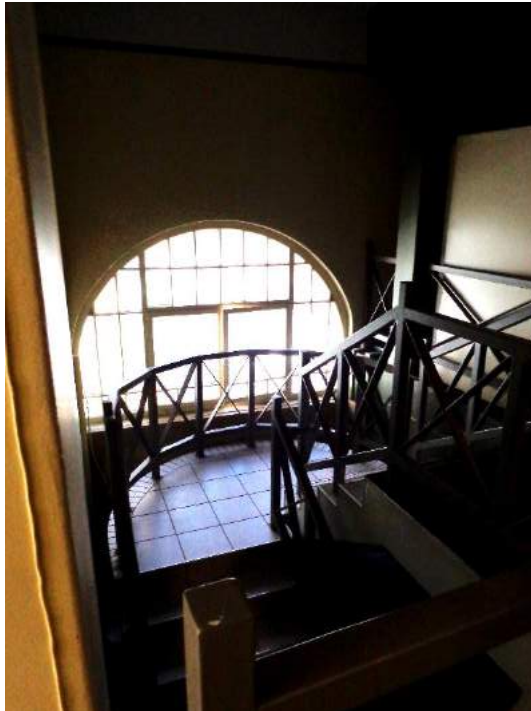
Figure 36 A new staircase replaced the original stage (photographs by author, 7 April 2017)
