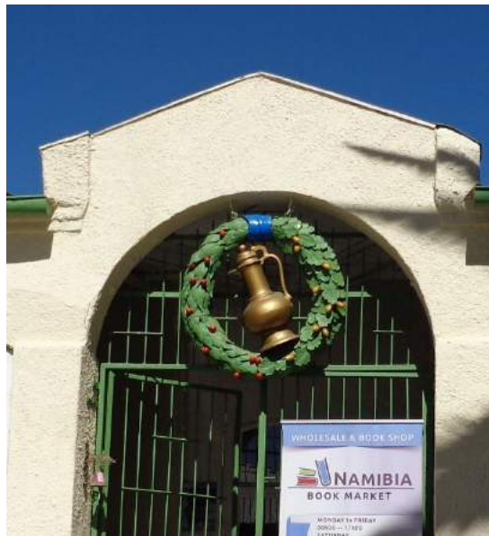
Figure 12 The Grüner Kranz (Green Wreath) sign hangs proudly above what used to be the entrance to the original hotel, now occupied by a bookshop (photograph by author, 21 July 2017)
