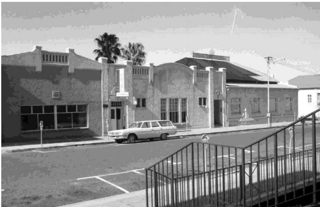
Figure 39 Front facade of Kaiserkrone complex on Post Street before it was pedestrianised (National Archives of Namibia: Edda Schoedder Collection)
