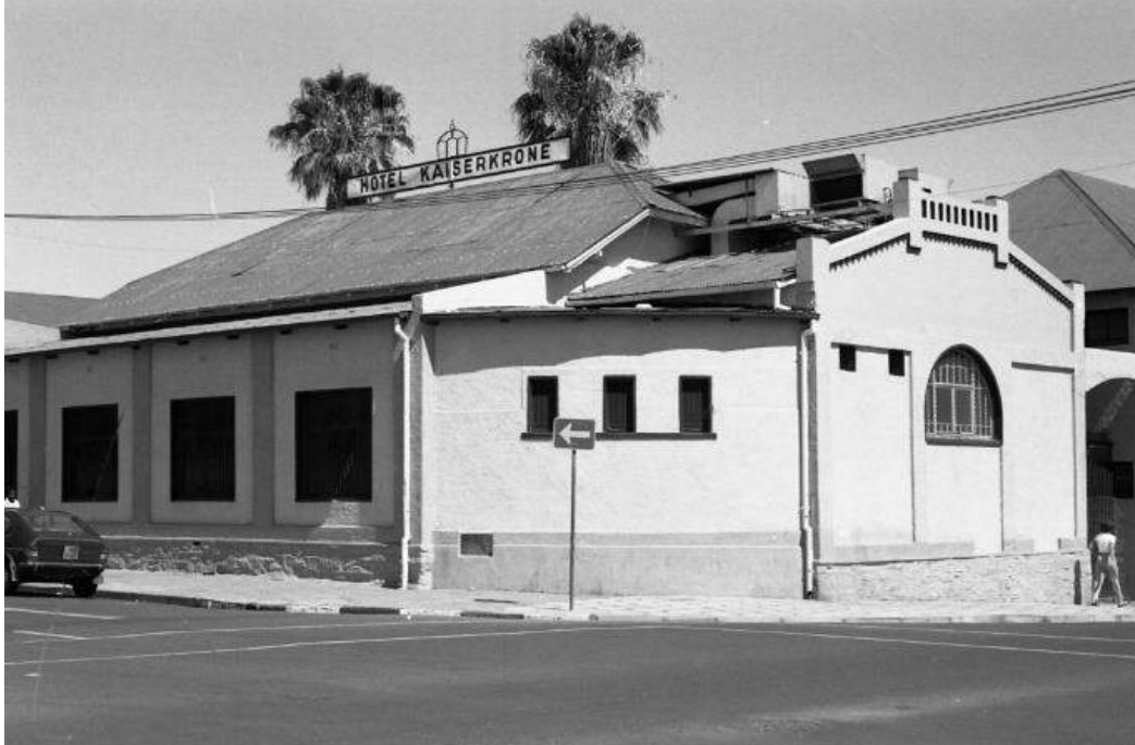
Figure 38 Corner of Kaiserkrone Hall on Post Street before it was pedestrianised (National Archives of Namibia: Edda Schoedder Collection)
