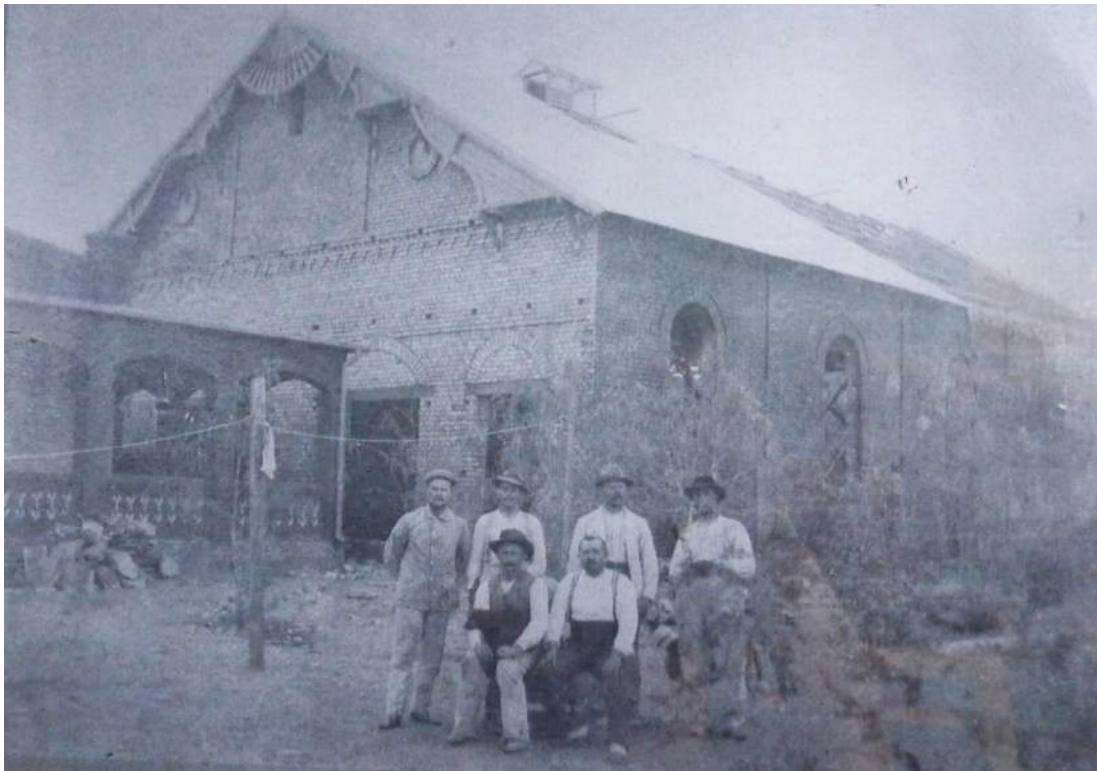
Figure 19 Brüsshaber (front right) and a small team of builders during the construction of the hall in 1906 - note the external decoration of the gable (Diener personal collection)
