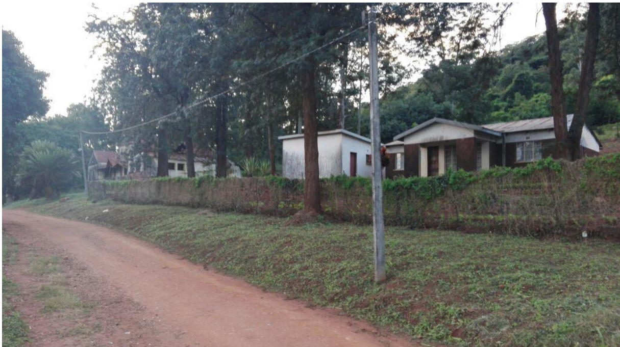
Figure 68: Current pastor's house opposite old parsonage on the far left (Source: Andani Ravhuanzwo, 2018).
