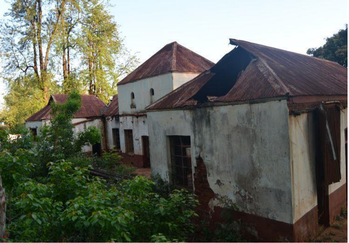
Figure 52: Bushy rear elevation of parsonage (Source: Author, 2017).
