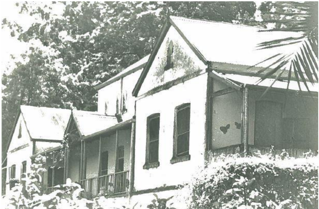
Figure 18: Rear elevation of parsonage in the 1940s (Source: Source: UNISA archives, Hesse Collection of German Africana Accession 89, Fobbe Photo Collection Part 1, No 34.34.2 Photo no. 109).
