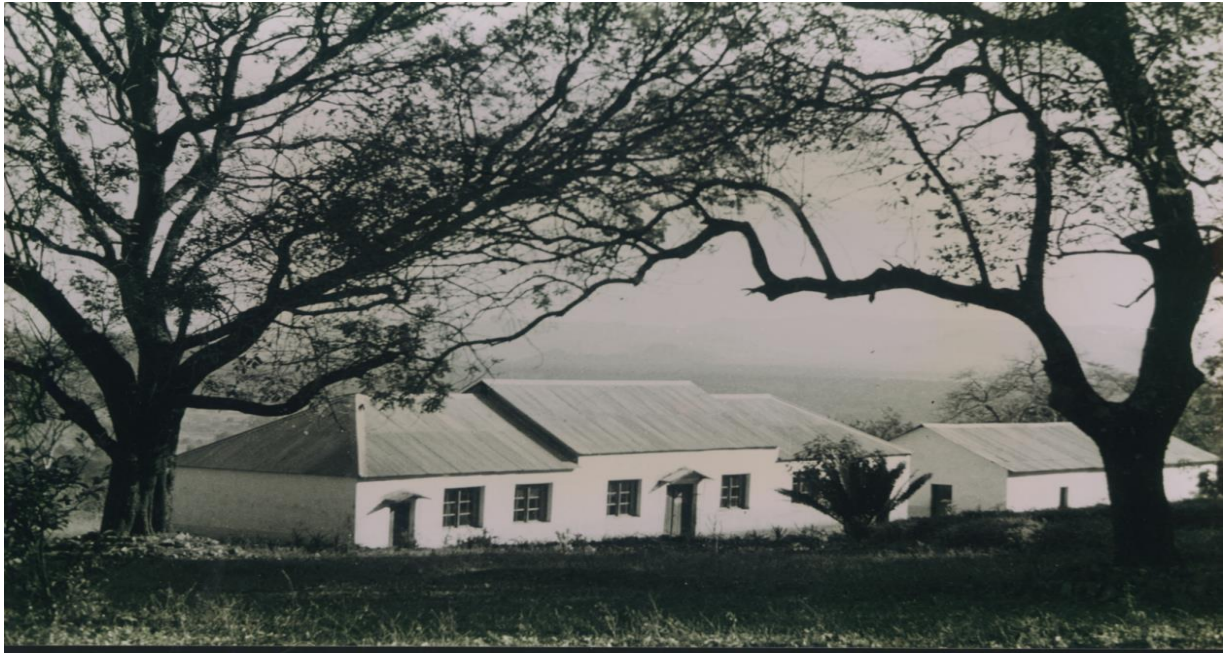
Figure 32: Georgenholtz Primary School with additional block in the 1950s (Source: Source: UNISA archives, Hesse Collection of German Africana Accession 89, Fobbe Photo Collection Part 1, No. 34.34.2, Photo no. 108).
