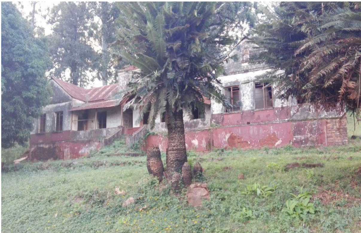
Figure 47: State of parsonage today (Source: Andani Ravhuanzwo, 2018).
