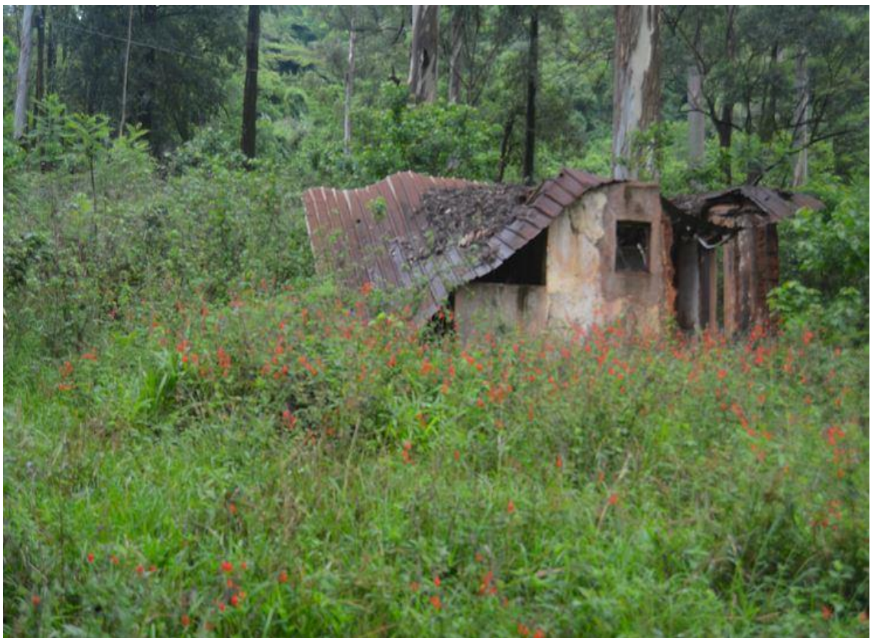
Figure 65: Dilapidated horse stable (Source: Author, 2017).
