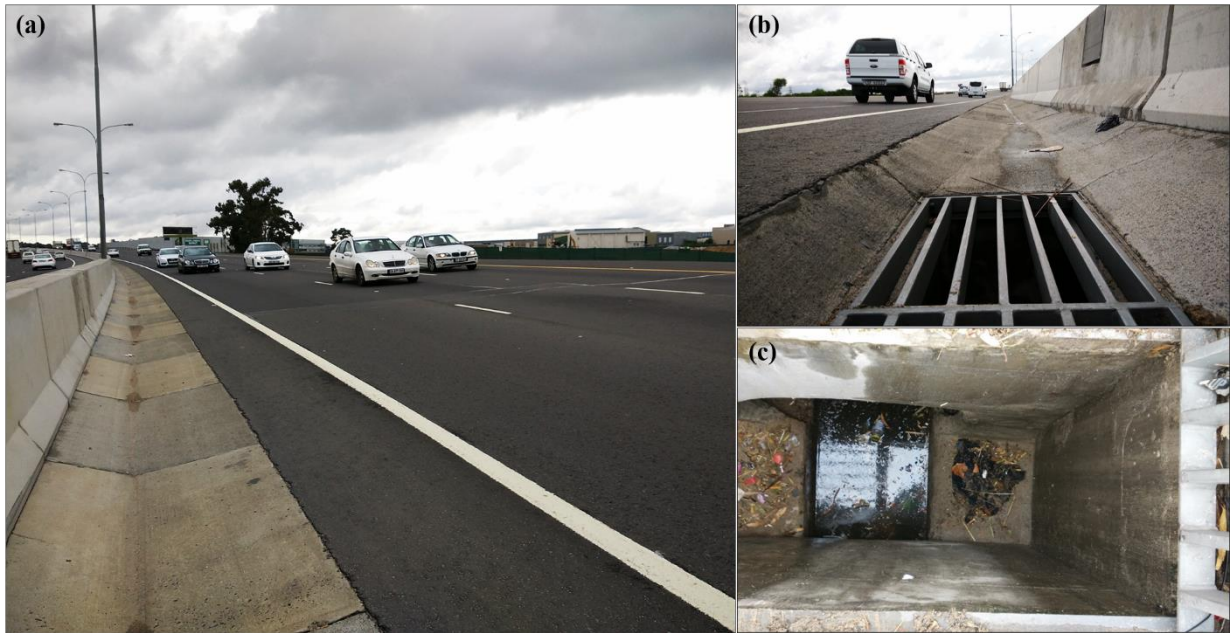
Figure 4-3: Sample Site 1 (a) the asphalt catchment area and concrete median drain, (b) concrete drain and catchpit inlet, and (c) plan view of the catchpit
