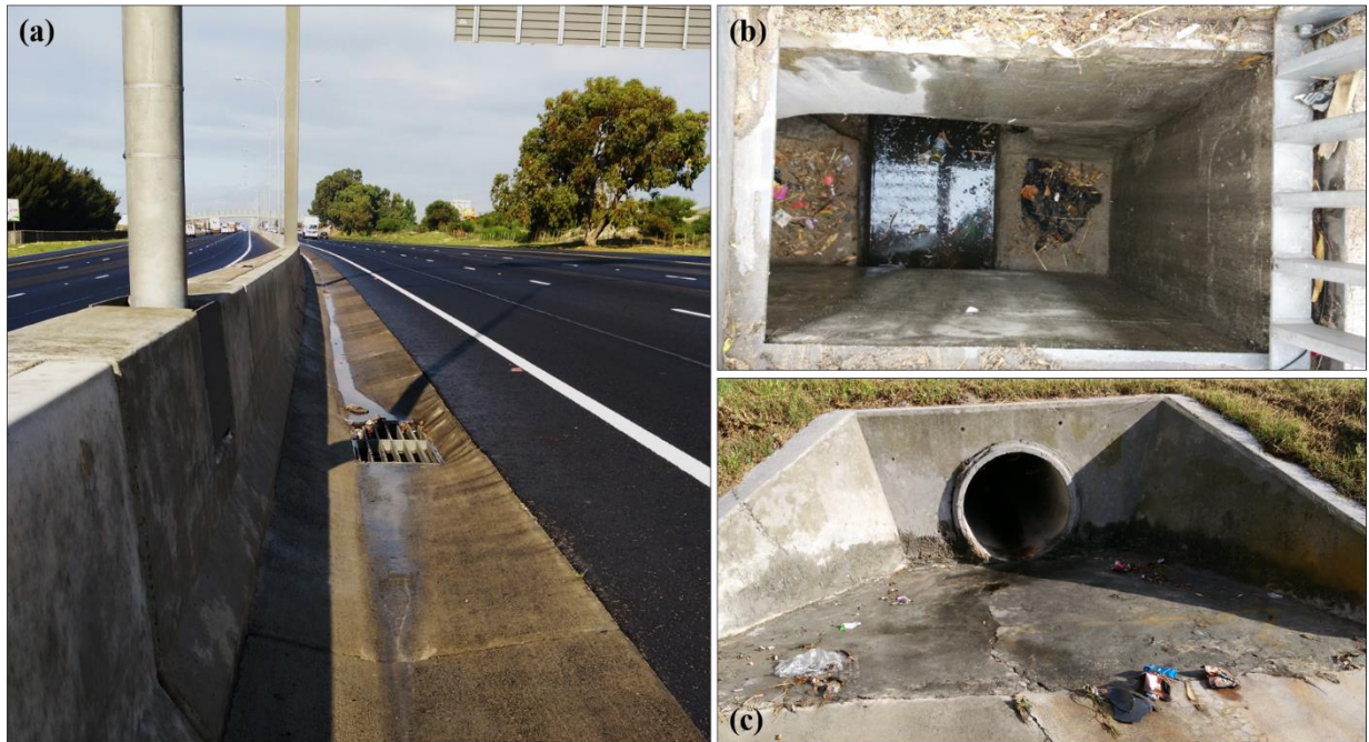
Figure 3-7: R300 road drainage structures where the road drains to the median: (a) a median surface drain, (b) catchpit plan view, and (c) outfall to the verge
