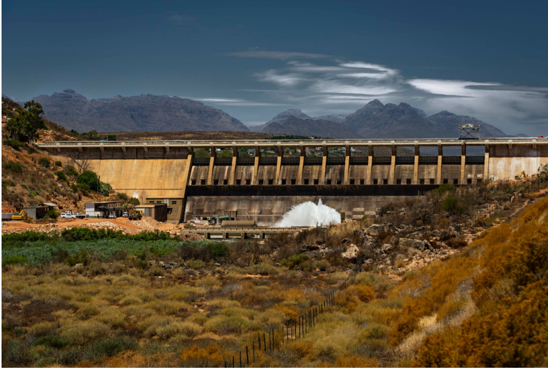
Figure 1.1. Clanwilliam Dam in January 2024. Photograph by Jeremy Shelton.
