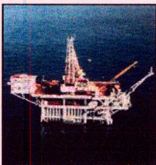
A typical offshore installation
