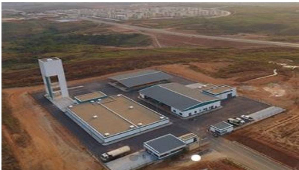
Figure 21: Water treatment plant
