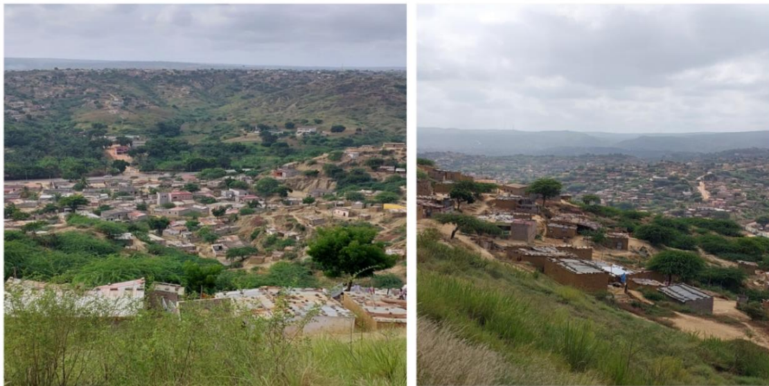
Figure 10: This image portrays Assaca neighbourhood and surrounding areas which are surrounded by natural elevations, from which water naturally flows downwards towards lower-lying regions and the variety of building materials used in the settlement.
