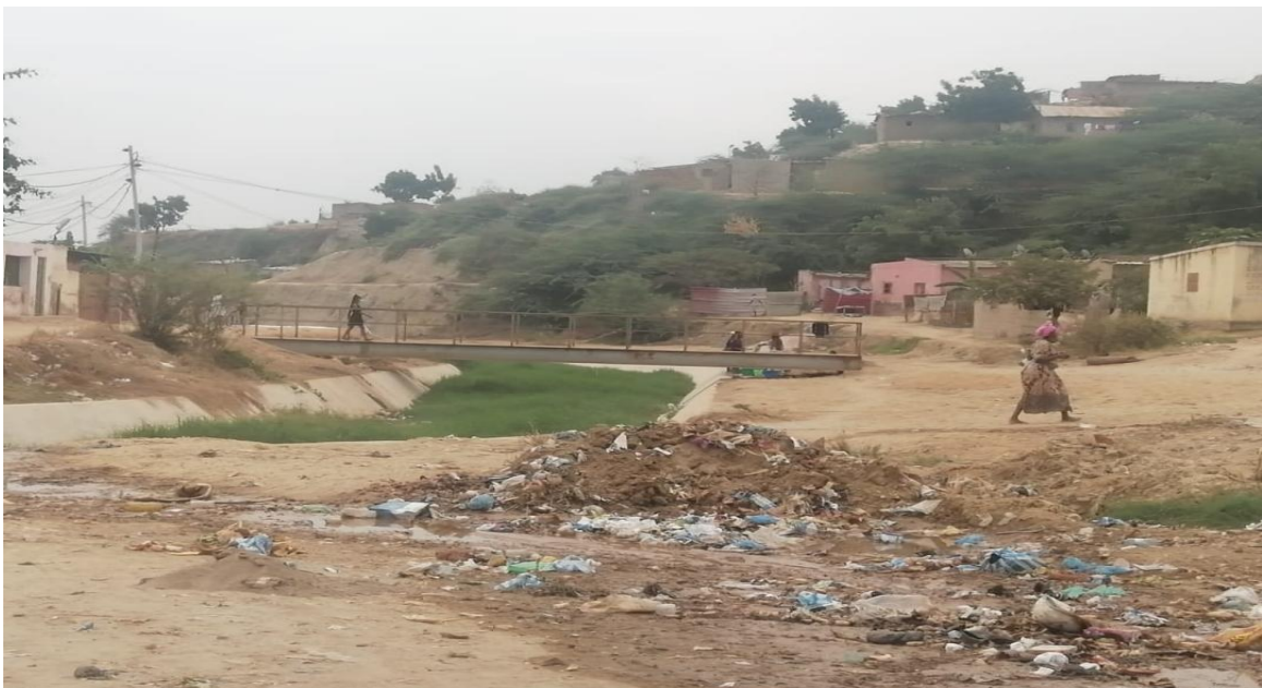
Figure 7: Drainage system in Assaca
