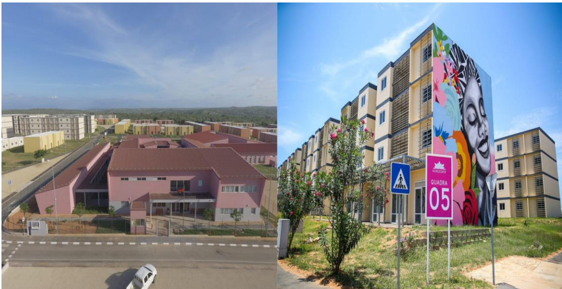
Figure 17: Paved roads and buildings in Kibaúla
