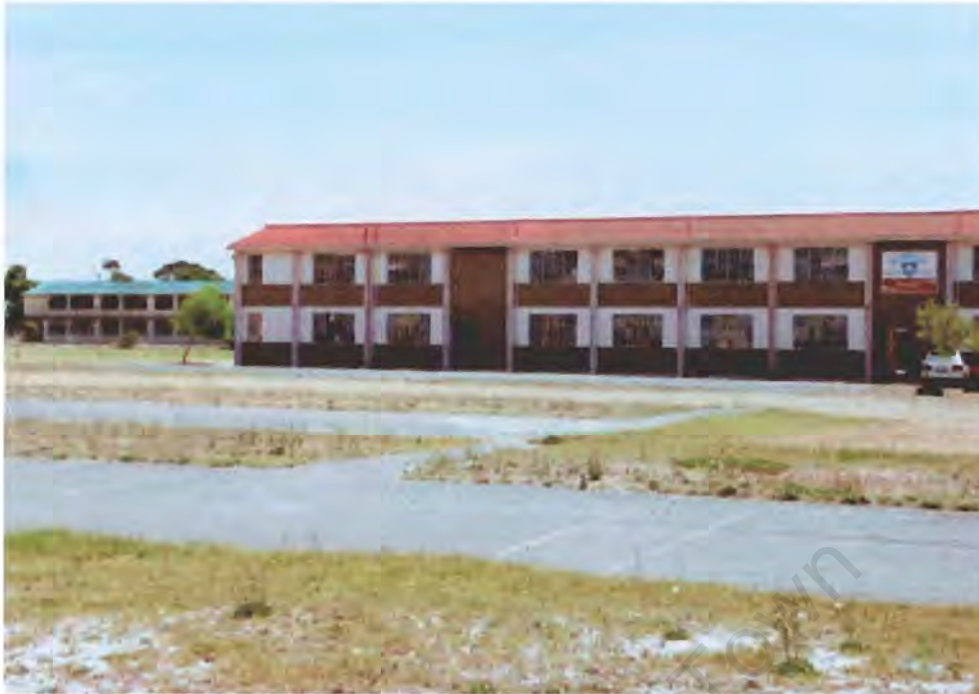
Photo 7 : Blomvlei Primary School
