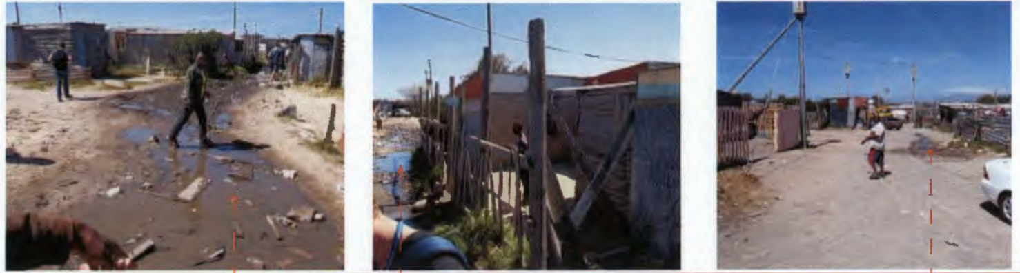
Fig 16 Uncompacted waste resulting in podding and the poor drainage of the soil means that during raining seasons flooding occurs here.
