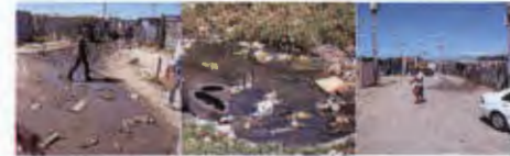
Unpermeated water seeping in building and the poor drainage of the site causes poor during raining seasons leaving visitors here.
