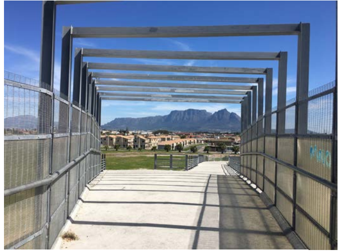
Fig.16 – Looking onto the site from the bridge
