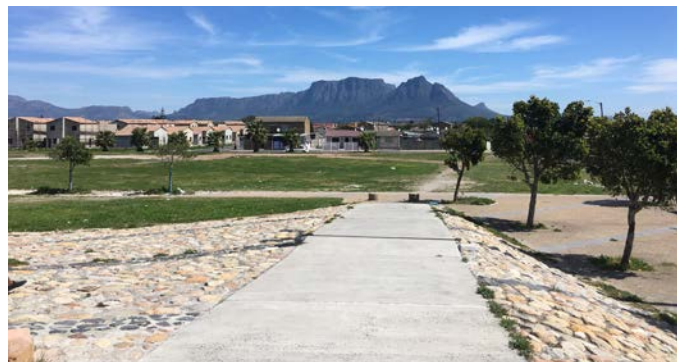
Fig.17 – Looking onto the site from the ramp
