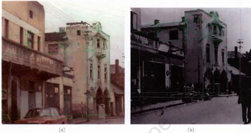
Figure 28: The two photographs of the British Bioscope, now with the reconstructed model projected onto them. The green lines are the edges of the model. Note how they conform closely to the original marked out lines (still partially visible in red).
