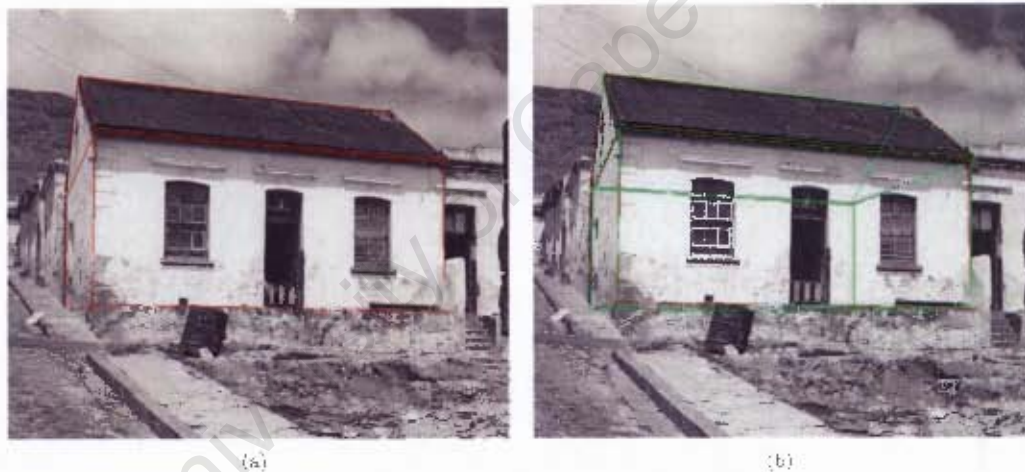
Figure 30: The single photograph used to reconstruct a small, District Six residence. (a) is the original input photograph, after the relevant edges have been marked out, while (b) is the photograph with the reconstructed model projected onto it from the perspective of the reconstructed camera. Note the error at the top right-hand corner of the roof.
