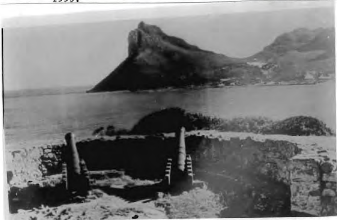
Fig. 210 Right gun traverse tracks, area F, ca 1930 (South African Library, PHA: Milit. Facilities).
