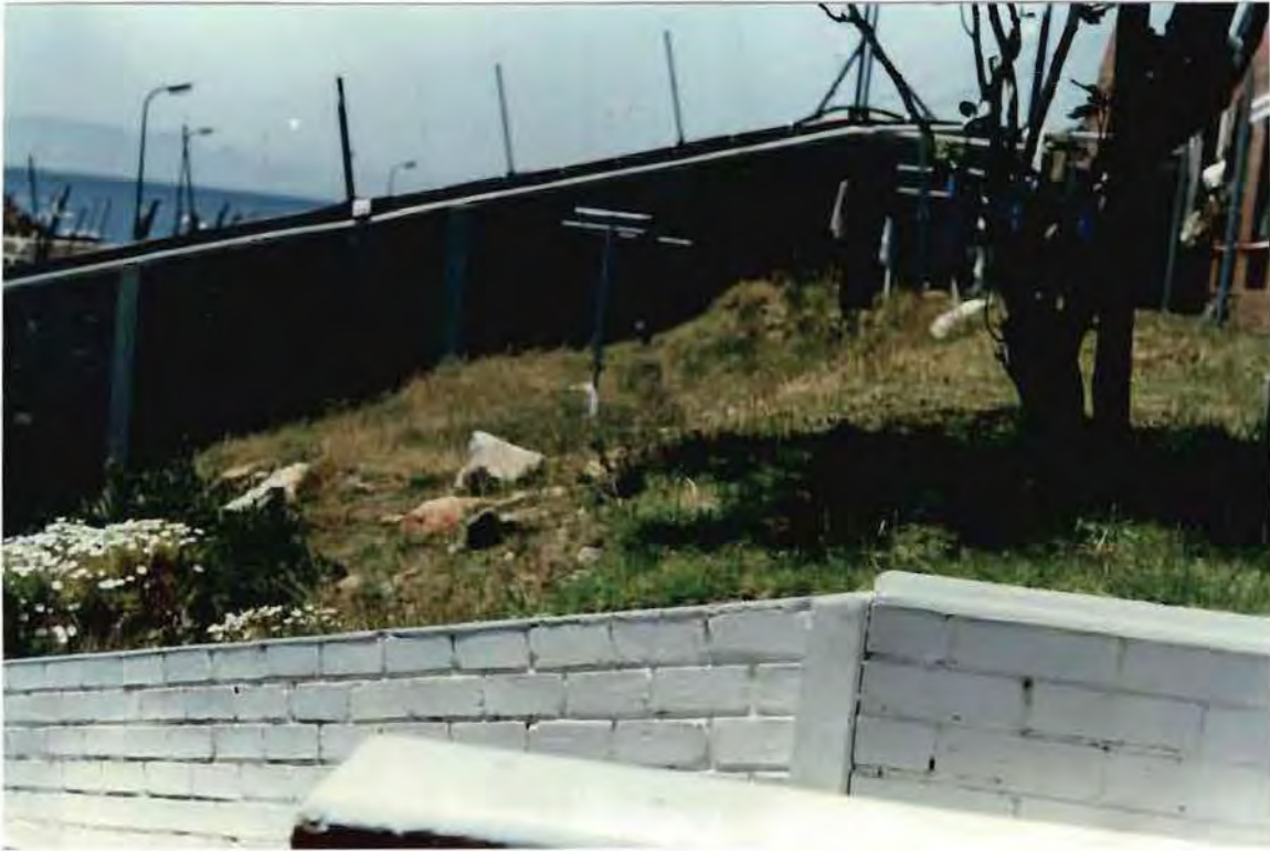
Fig. 100 Rampart wall of the South Battery, 1993.
