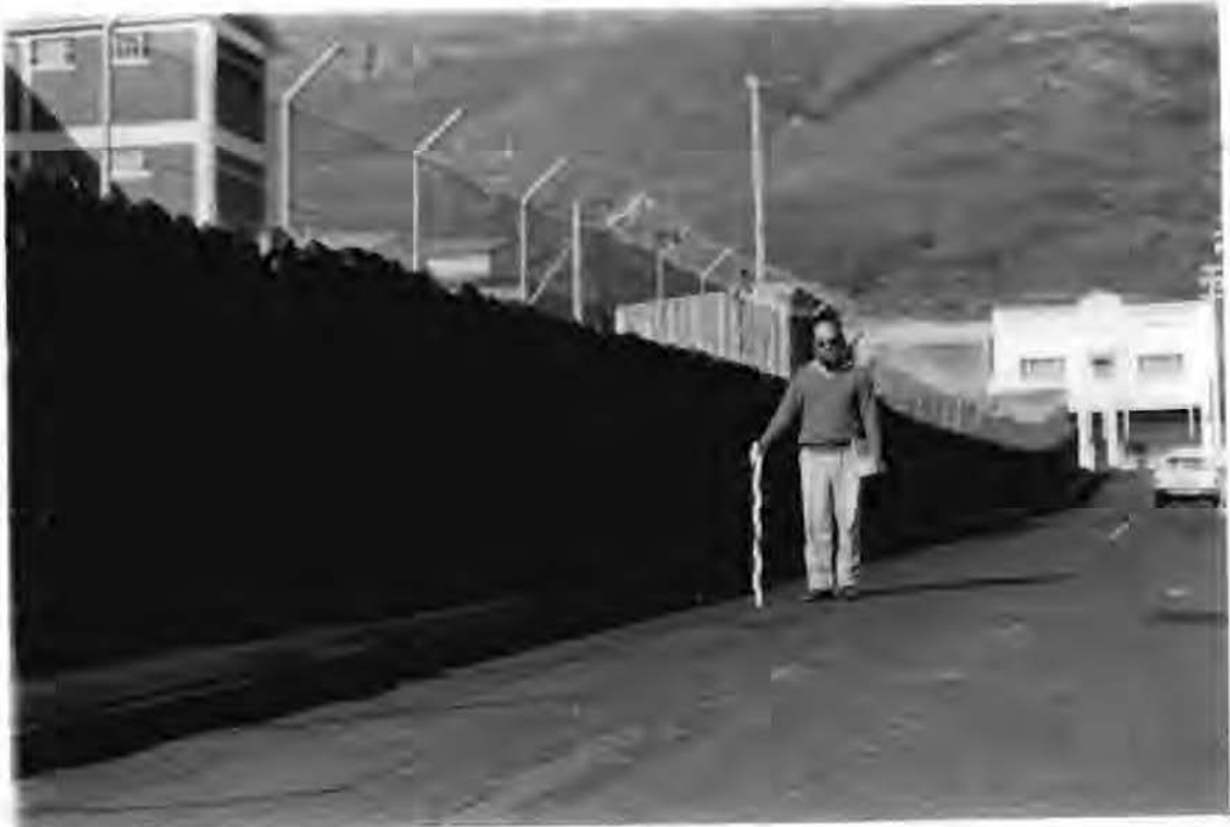
Fig. 256 Remains of a wall, encompassing the French Lines near the Hollands Redoubt, Woodstock, Cape Town, 1993.
