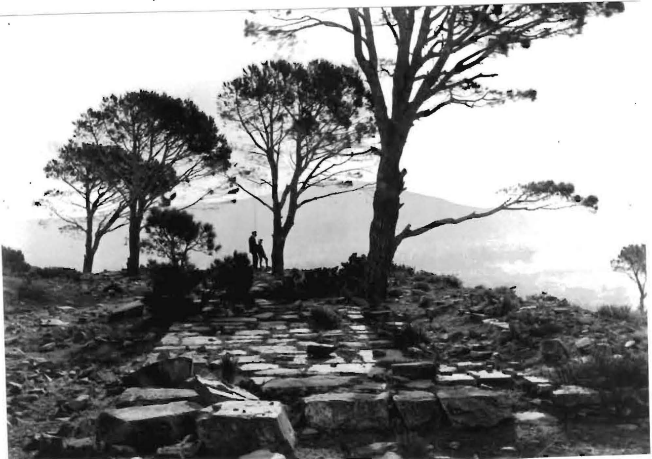
Fig. 73 Cradock Battery, ca 1920 (Cape Archives, M822).
