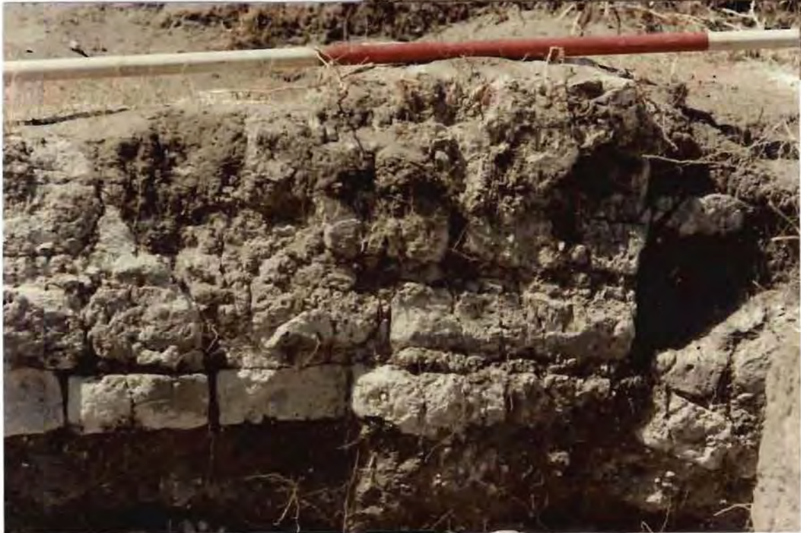
Fig. 181 Lining of the embrazure walls with lime/cement bricks.
