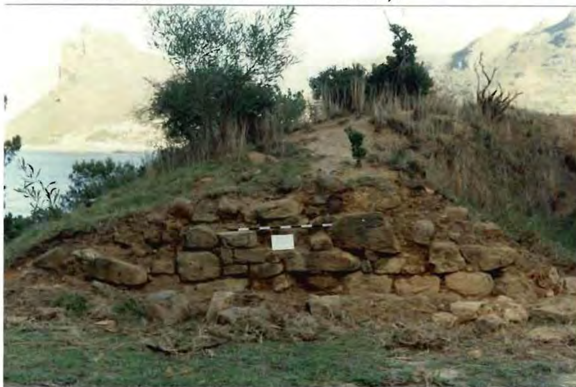
Fig. 206 Retention wall of the middle level rampart, area E, 1993.
