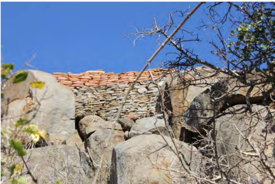
Figure 34: Retaining wall on eastern side of Mapela
