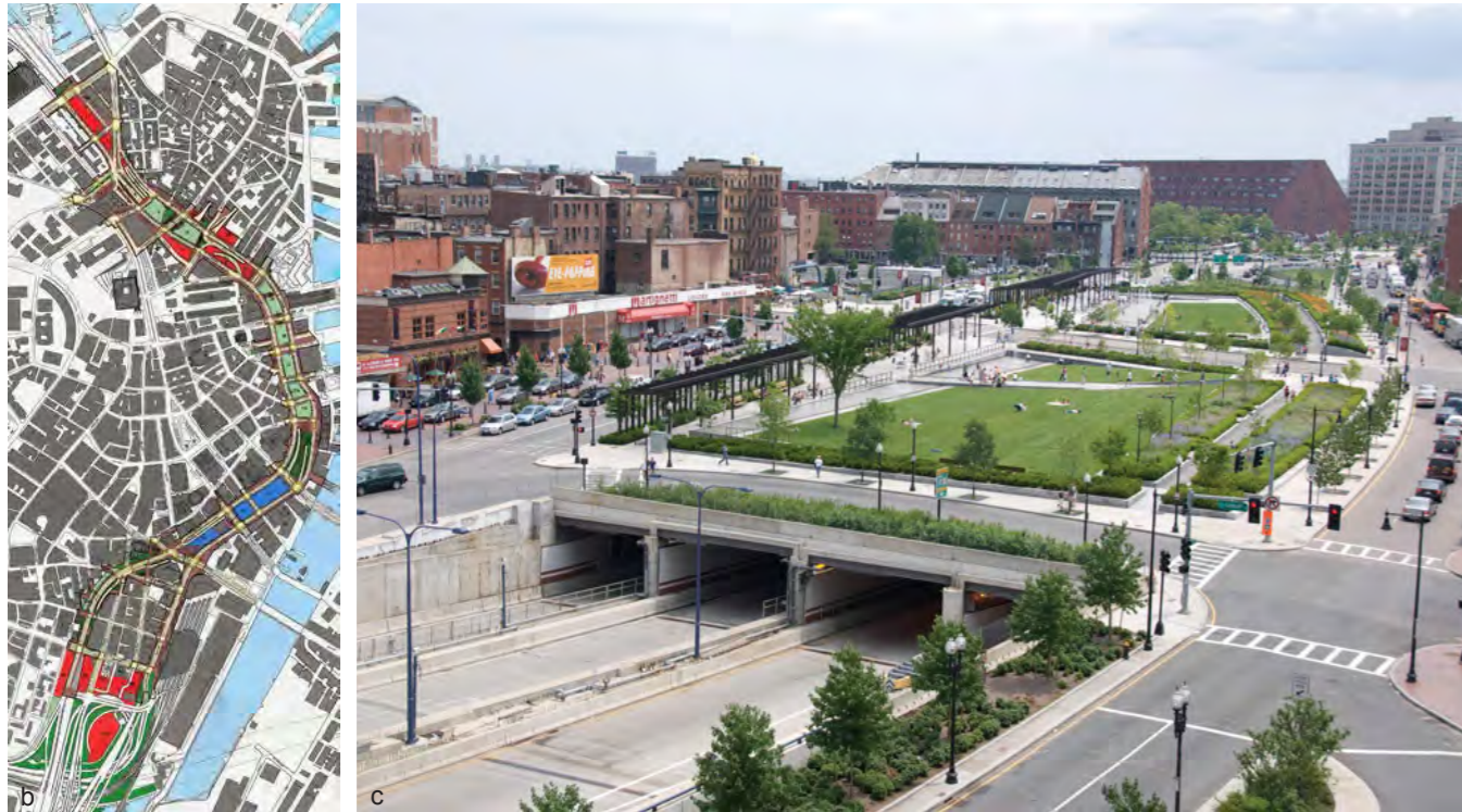
fig. 15 before and after; stitching together the divided urban fabric; new green public space in the city
