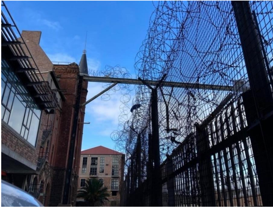
Figure 19: Parapets and fences covered in barbed wire fencing at the Woodstock Brewery, Beach Road.
