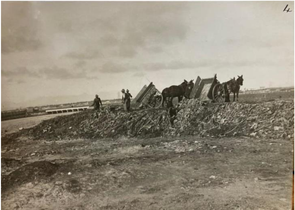
Figures 37 & 38: Kelp removed from Woodstock Beach offloaded at Salt River dump.
