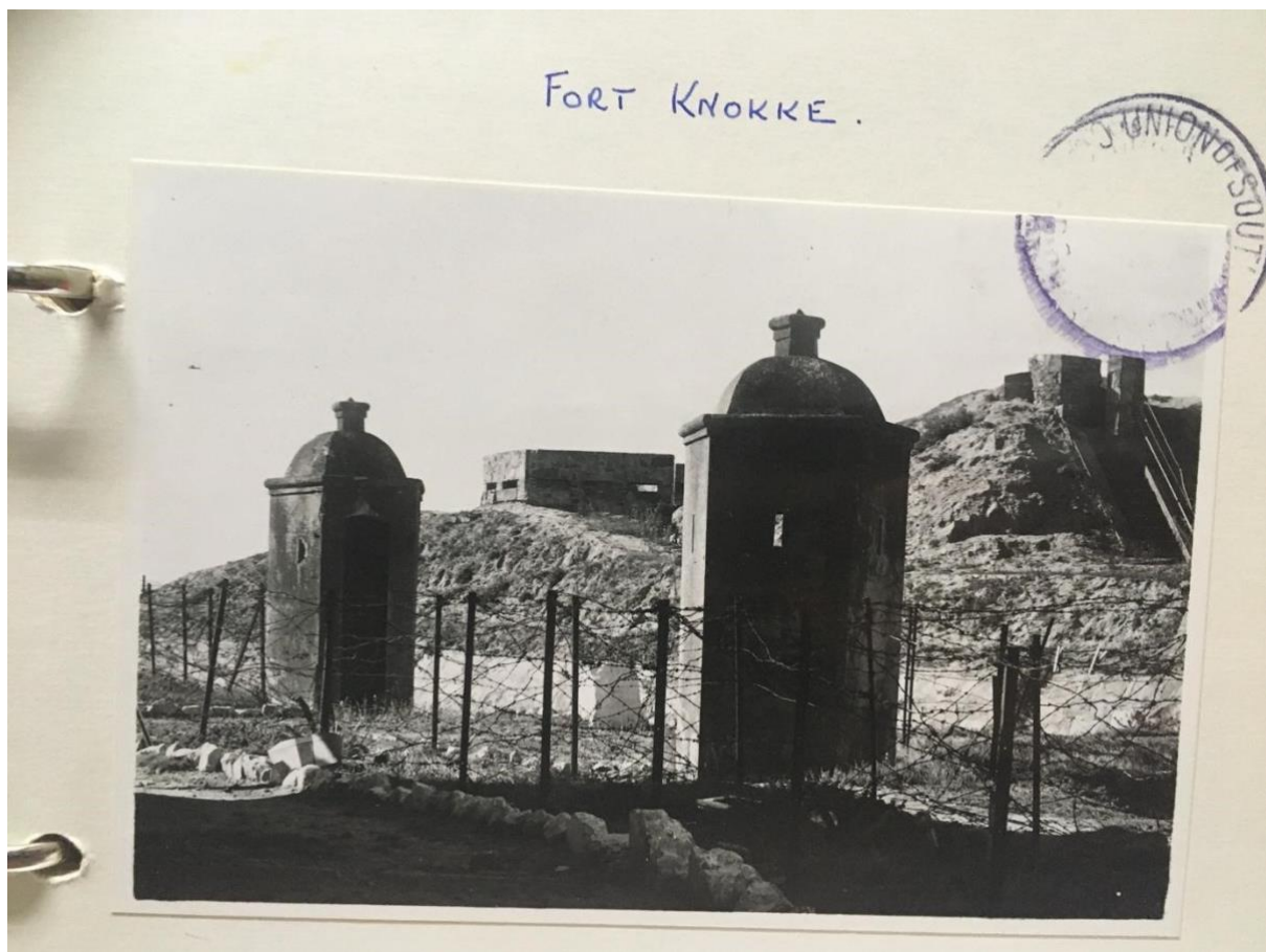
Figure 16: Black and white photograph of Fort Knokke on Woodstock Beach with fencing in foreground.
