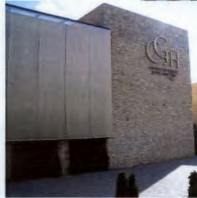
Fig 42 Hotel Golf y Spa Castillo de Gorraiz, Gorraiz, Spain by Iribarren, Rojas, Valls, Zabala. resource: www.diedrahtweber.com accessed 2 May 2010
