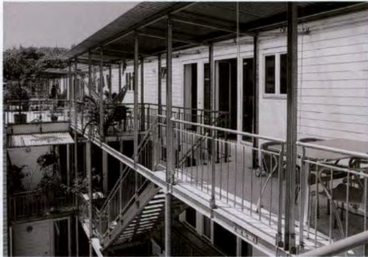
Fig 5: external balconies of Hellmustrasse by ADP in Zurich, circulation made generous to allow for more uses and occupation and not merely a means of access from one level to the next. resource: Till, J. 2008,29
