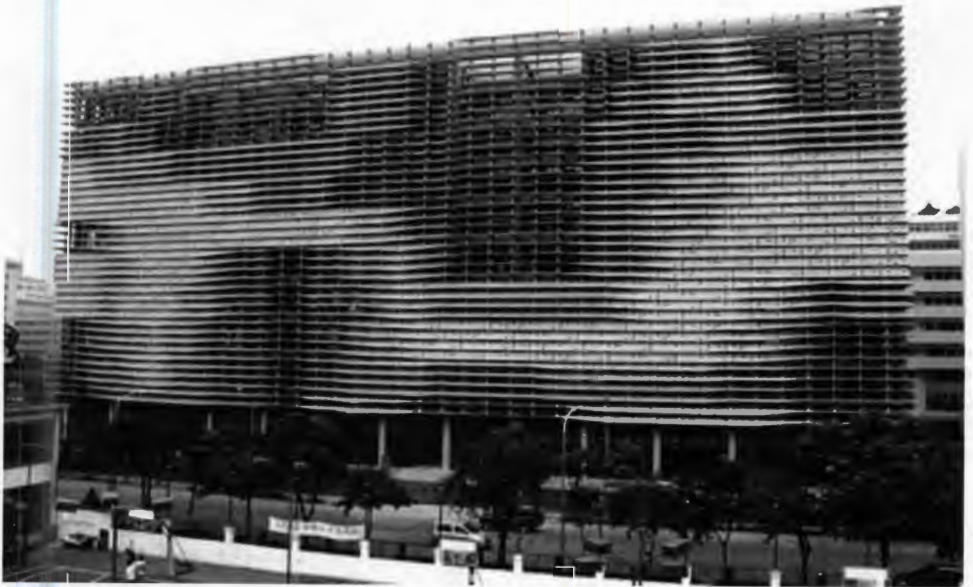
Fig 4): Hadighi designed a woven concrete facade for the Skantou, China headquarters for Lafayette 148, a New York-based clothing designer and producer. Image courtesy Studio for Architecture. (resource: www.architecture.uark.edu accessed 14 may 2010) The façade has a textile like quality although a very Architectural material- concrete is employed.
