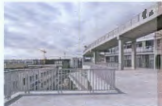
The large roof top that can be used for major events
