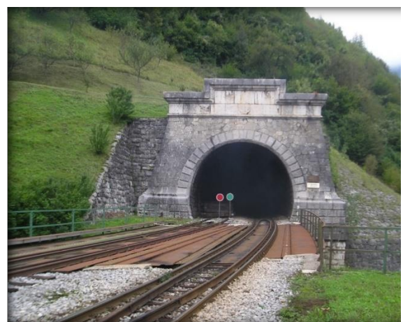
Figure 1-4: Rail Tunnel External View
