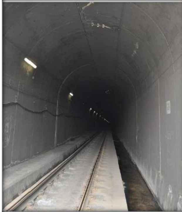
Figure 2-13: Railway Tunnel Internal View (Gräbe & Fröhling, 2017)
