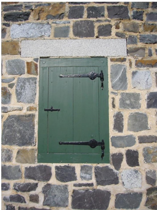
Figure 9: Corporal's House: Detail of new copy of window/shutter, iron-mongery and granite lintel; (Photo: Author, 2010)
