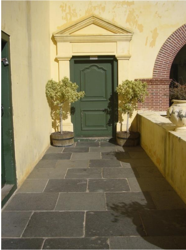
Figure 27: Pool Complex: Front door detail with pilasters and pediment; (Photo: Author, 2010)
