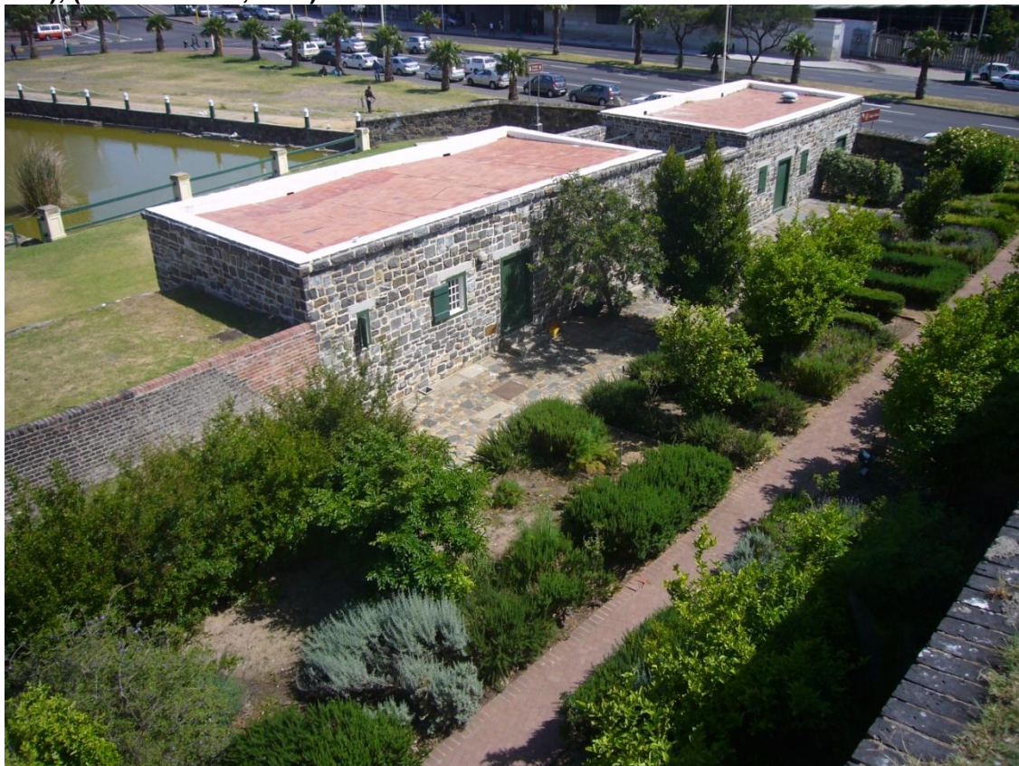
Figure 7: Corporal's House: Contemporary view onto east elevation from Buuren Bastion; with refilled moat in back; (Photo: Author, 2010)
