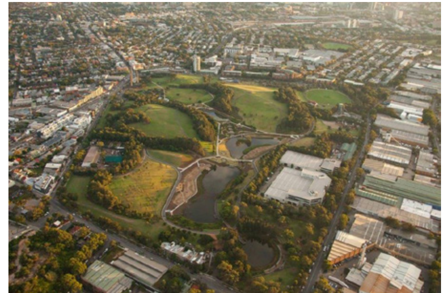
Sydney, Australia: Stormwater re-use park (Turf Landscape Architects) integrates engineering and water sensitive urban design to capture and filter stormwater from the surrounding area (Image Source: http://turfdesign.com/sydney-park-water-re-use-project/ )
