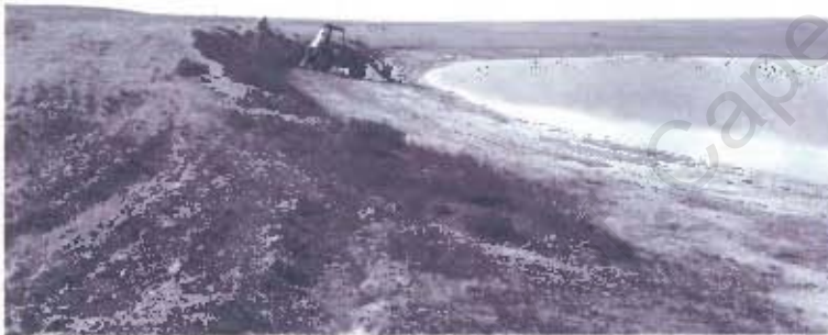
Figure 5.4: Back-hoe excavating lunette face. Furrowed fields in foreground. View facing eastwards (SMG, 4 June 2002).
