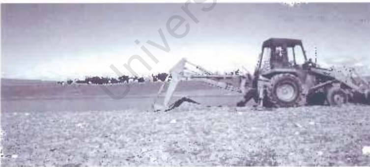
Figure 5.5: Back-hoe excavating lunette crest. Photo facing south, across the pan to the Basson farmhouse (SMG, 4 June 2002).
