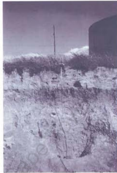
Figure 5.9: Photograph of the south side of the gully sampled at Voelvlei (profile VL) . (SMG, 5 October 2001).
