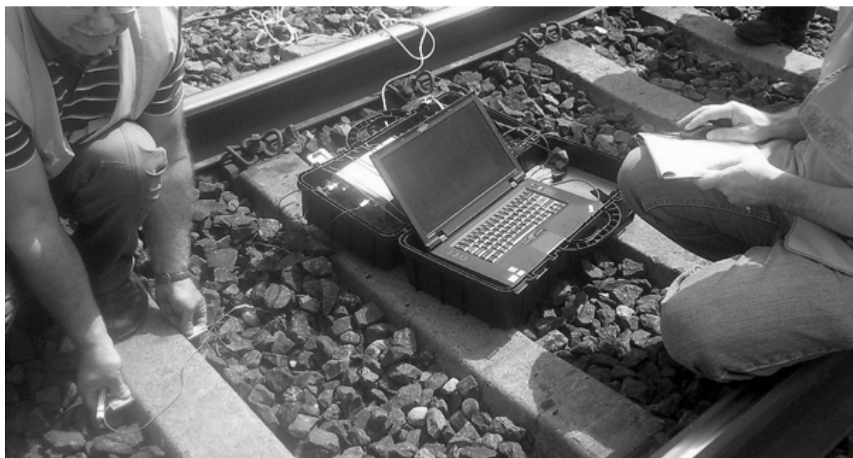
Figure 2-33: Sleeper Testing on Latvian Railways using Ultrasonic Equipment from Riga University (Tatarinova et al., 2018)
