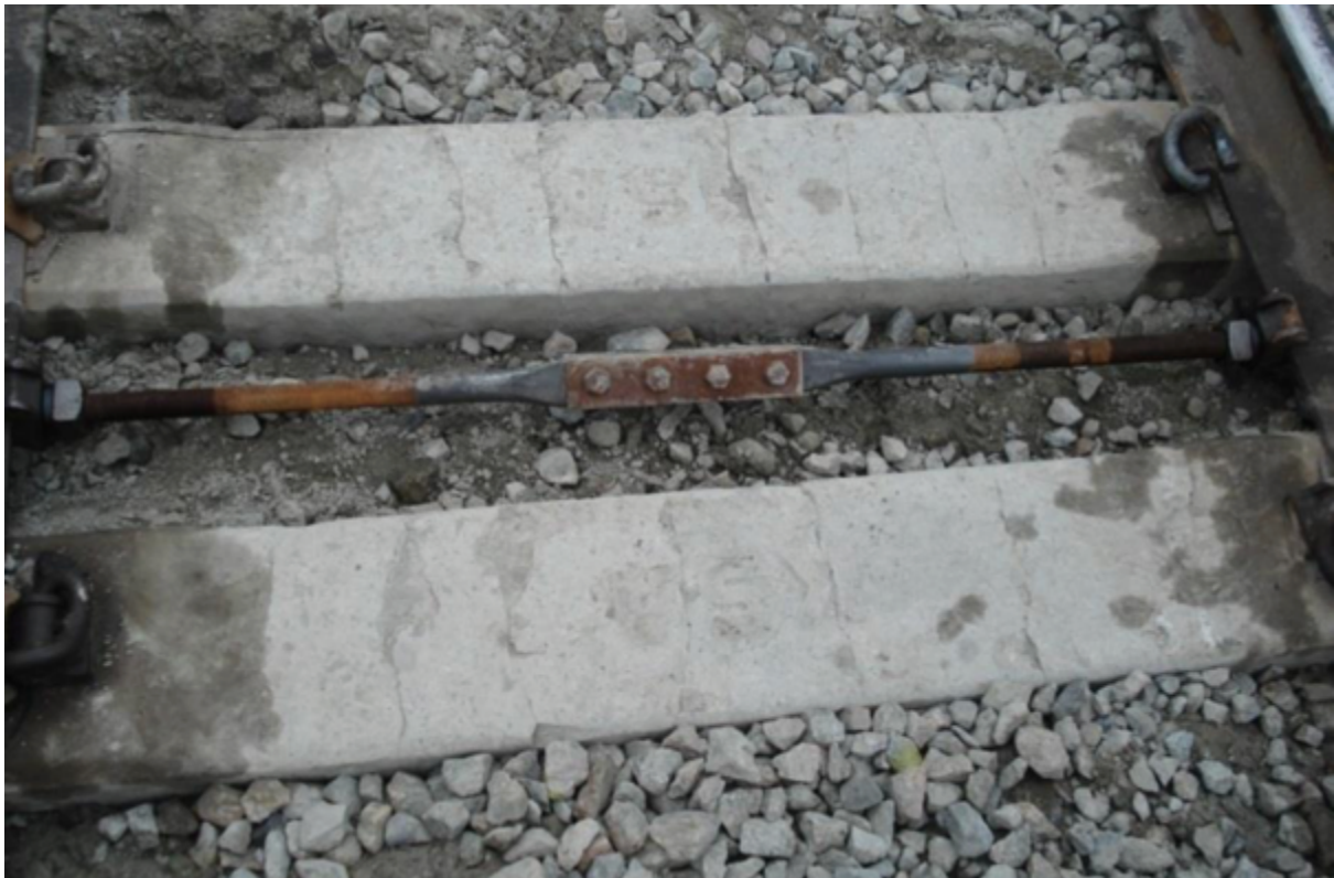
Figure 2-18: Example of Centre Binding of Concrete sleepers (NTSB, 2014)
