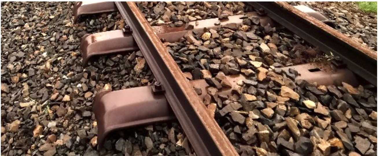
Figure 2-6: Example of Steel Sleeper with Exposed Shoulder (Photo by Author)
