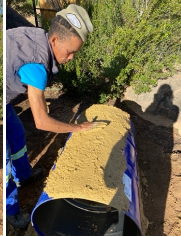
Figure 11: Building layers on top of the drum
