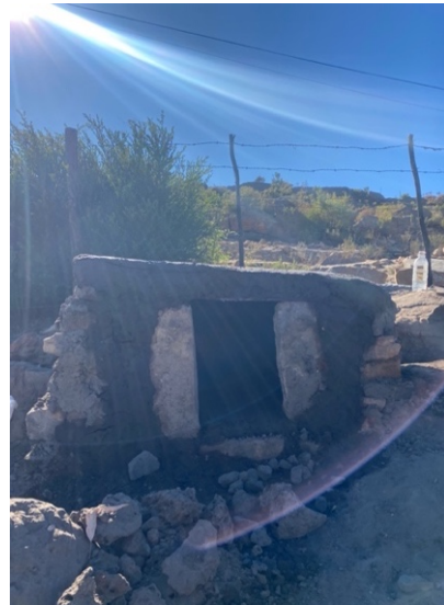
Figure 16: Outdoor oven made from clay and stones at Menskraal
