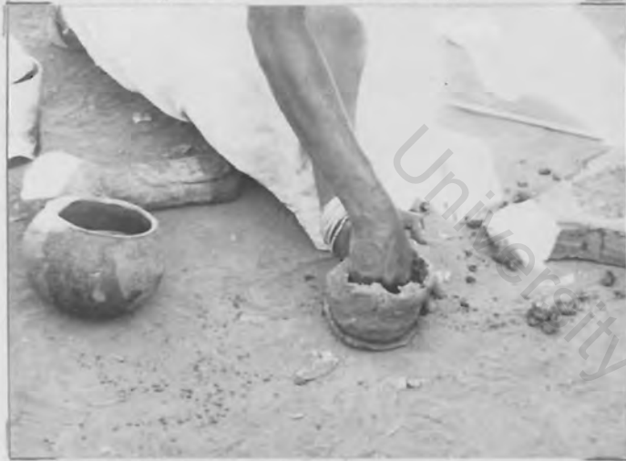
NO. 61 Hollowing the lump.
