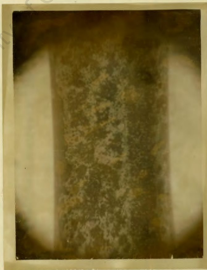
Plate 22. Corroded Metal Surface. x 2
