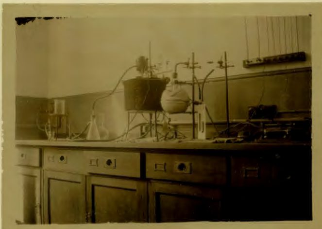
Plate 1. First Corrosion Test Apparatus.
