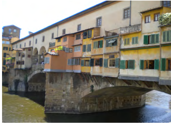
Figure 13 - Ponte Vecchio. The ground floor shops and living areas above are 'clipped' onto the side of the bridge, and the Vasari Corridor, inaccessible to the public runs along the upper most level.
