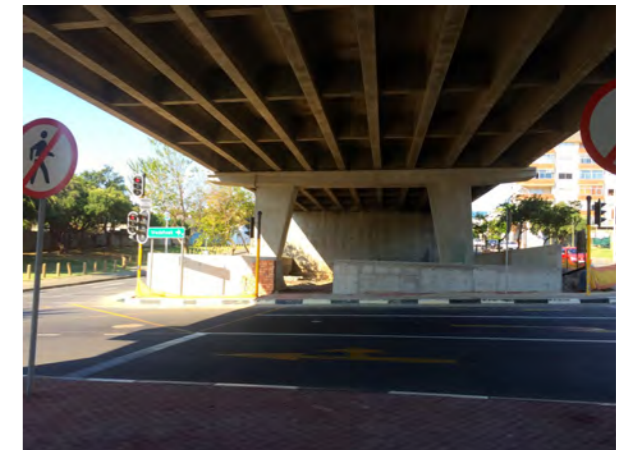
Figure 23 - Image of the residual space underneath the highway (before).
