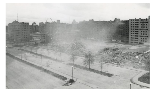
Figure 1. The second widely televised demolition of a Pruitt-Igoe building in 1972.
