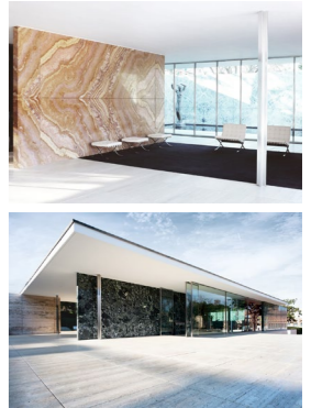
Figure 99. The golden onyx marble above, and the ancient green marble from Greece below. Note how important a role these marble edifices play in the structure.
