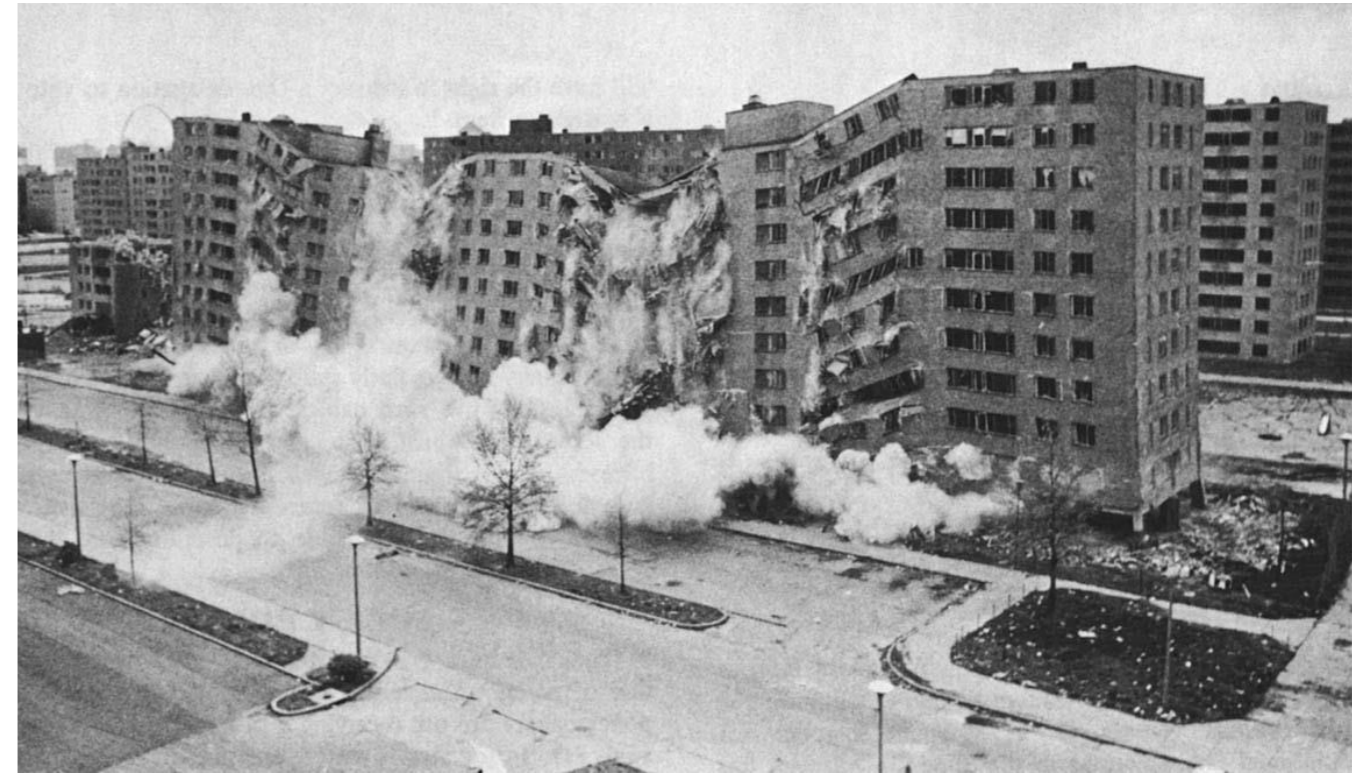
Figure 18. The second stage of demolition in April 1972.
