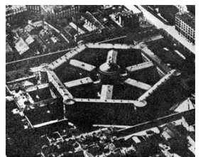
Figure 71. Prison de la Petite Roquette, Paris, built between 1825 and 1836 by Hippolyte Labas according to Jeremy Bentham's designs for the Panopticon. The structure was demolished in 1974.
