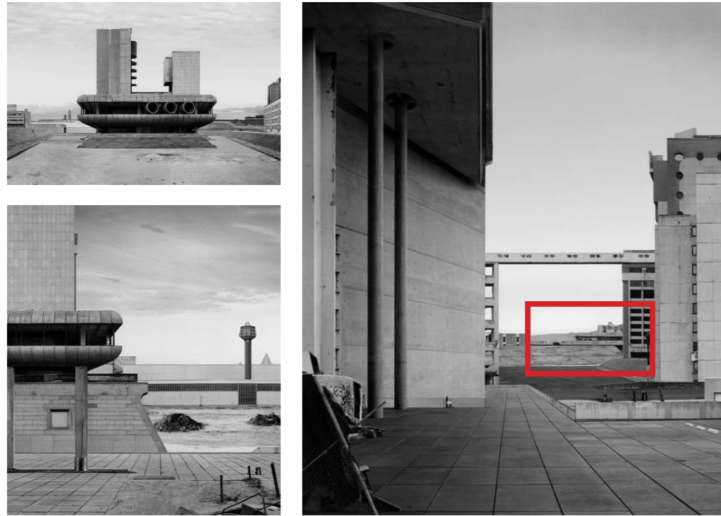
Figure 95. Notice how the same structural elements are repeated across S#13 , S#14 , and S#16 .
