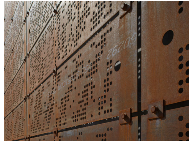
Figure 66 : Forsyning Helsingør Power Plant – Exterior detail [top left] (SSAB, 2018)
