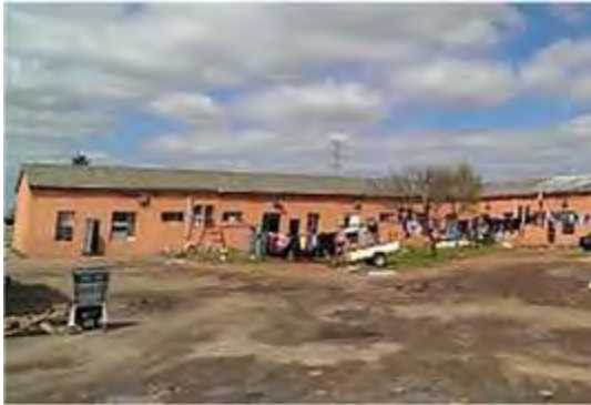
Fig.13 The 1925 Single Quarters (Main) Barracks, SAHRA "Grade I", (R.Smith, 2013)
