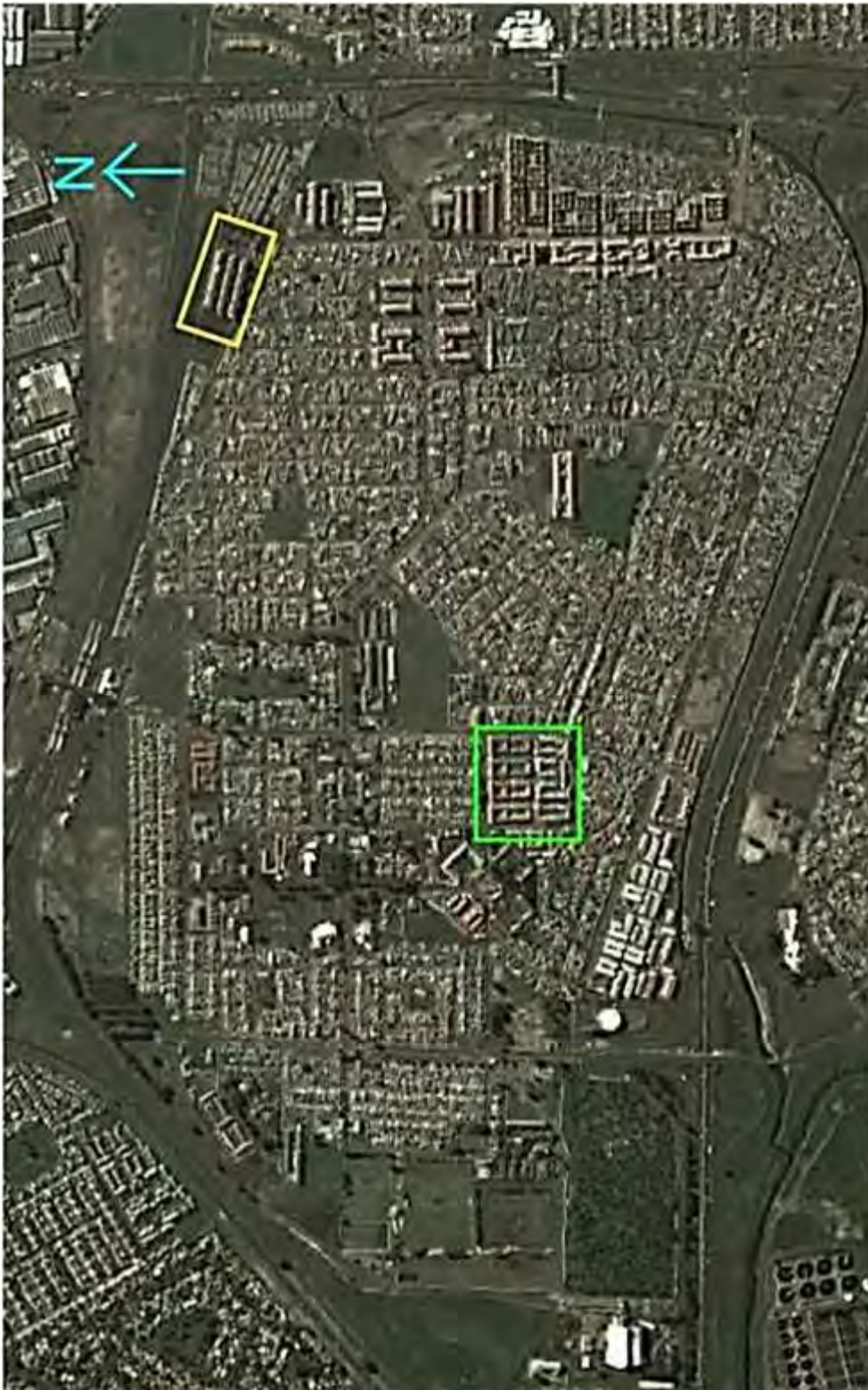
Fig.9 Aerial photograph showing the single quarters referred to as the “New Flats”, see green square, were constructed during 1970’s at the same time that the Railway Flats, see yellow rectangle, were built and station upgraded. (Google earth, 2013).
