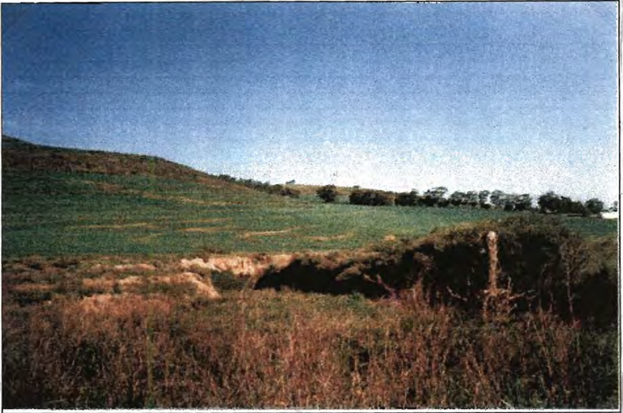
Figure 5.5b): A similar slope with an old gully at the bottom indicating erosion from years past, but the contour walls preventing further gullies from forming can clearly be seen in the background on the slope in 1994. The areas of light soil visible at the bottom of each contour wall show a new form of soil erosion resulting from the contour walls.
