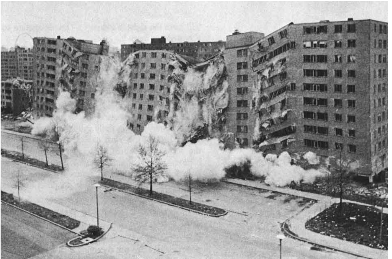
25 : The demolition of Pruitt Igoe
