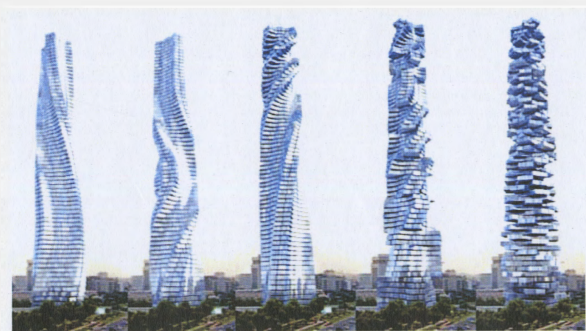
Fig. 2.19 The Dynamic Tower is a building that has the ability to rotate 360 degrees with individually controlled floors.
