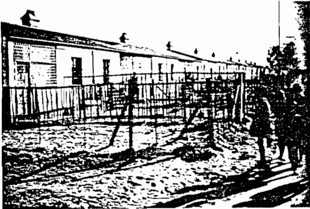
A ROW OF HOUSES IN THE 'OLD LOCATION'. THE FIRST HOUSE HAS A 'TRELLISED' VERANDAH.
