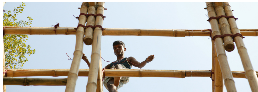
Figure 17 METI school, 2006 illustrating the jute rope lashing joint
