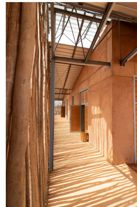
Figures 19 & 20 eucalyptus poles utilised as cladding for the facade, supported by steel structure
