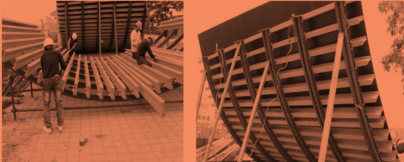
Figures 37 & 38 illustrating the making of formwork for the casting of a curved concrete element.
