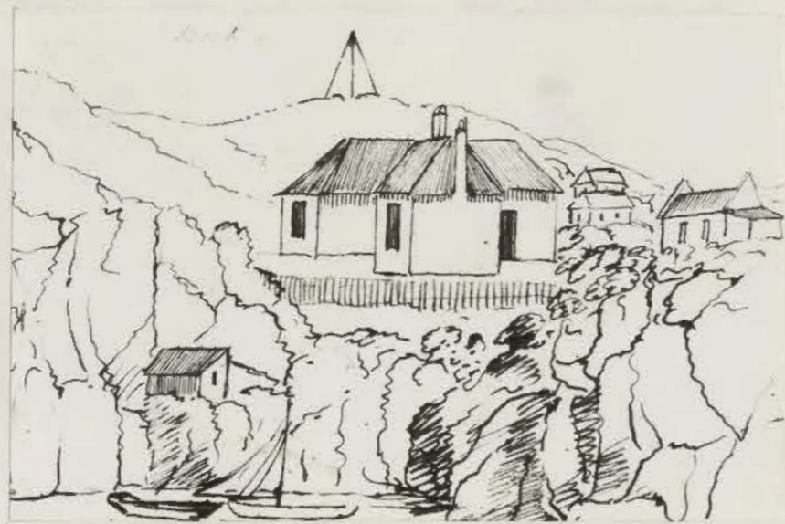
1. 'Craig Cottage' by S.E. Hudson (c.1822) showing Donkin's memorial to his wife. The buildings are probably those of the original military encampment. (Archives).
