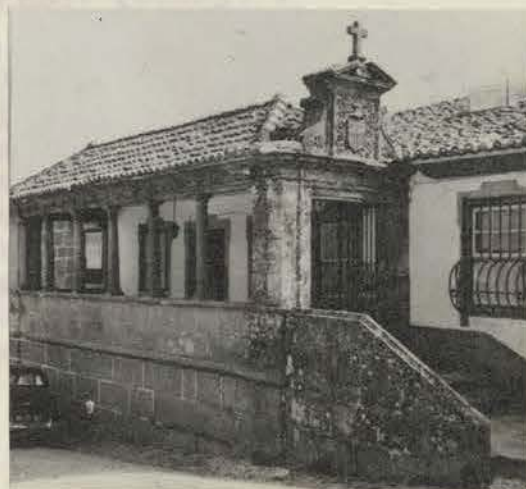
2C. 'Varanda' of a 'solar' at Guarda.
