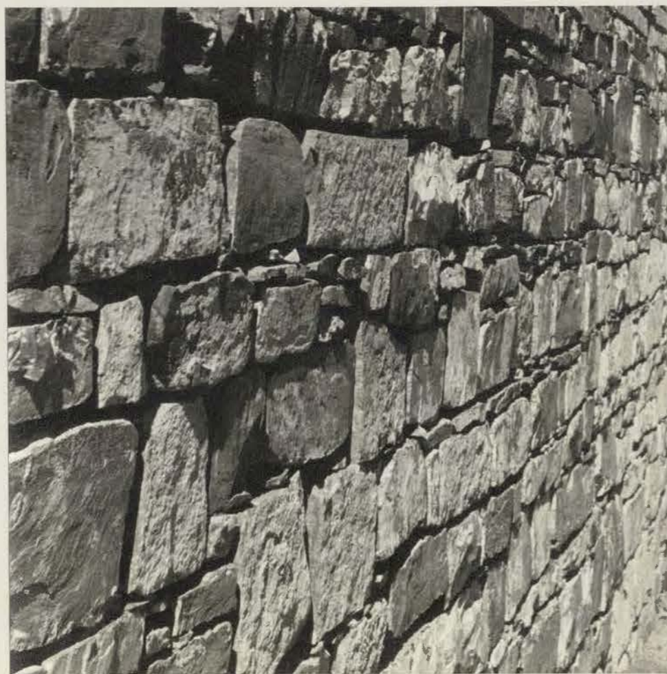
49. Squared coursed rubble stonework, Cradock.
