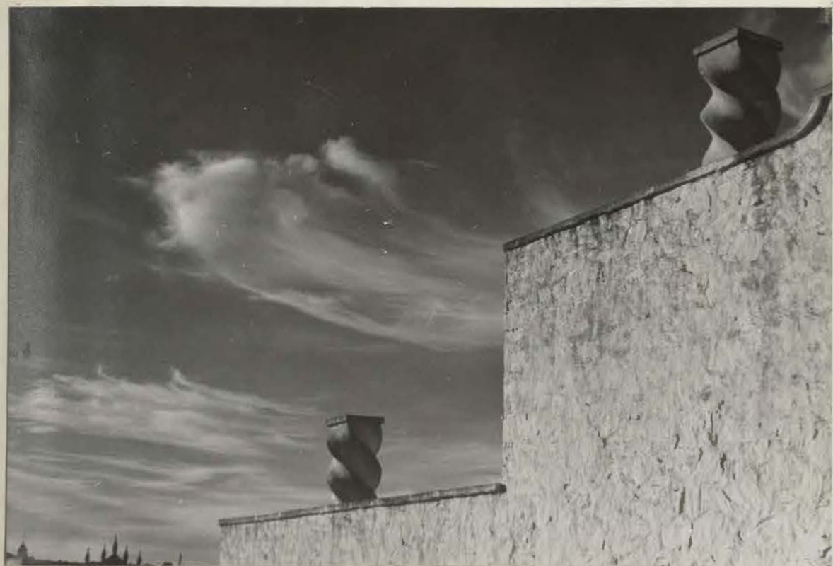
56. Spiral chimneys on a house in Beaufort Street, Grahams- town, which has a strong eighteenth century character, in spite of its exposed stone walls.
