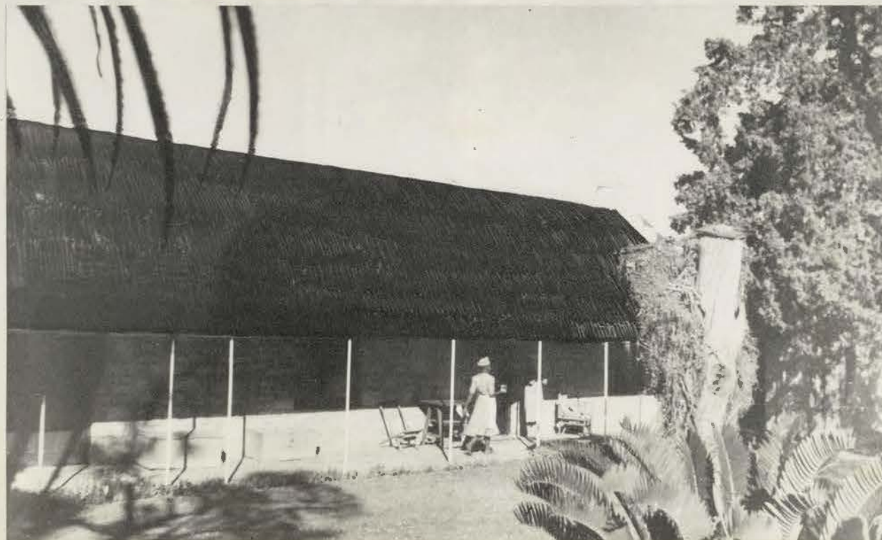
81. 'Assegai Bush'. The original thatch roof has been suggested in the photograph.
