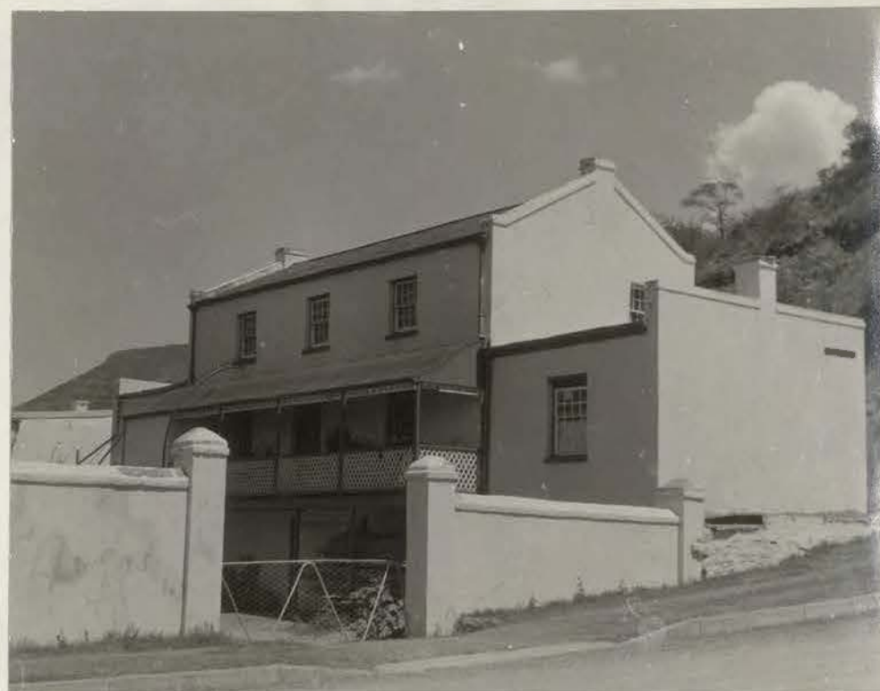
122. Old Mill-house, south side.
