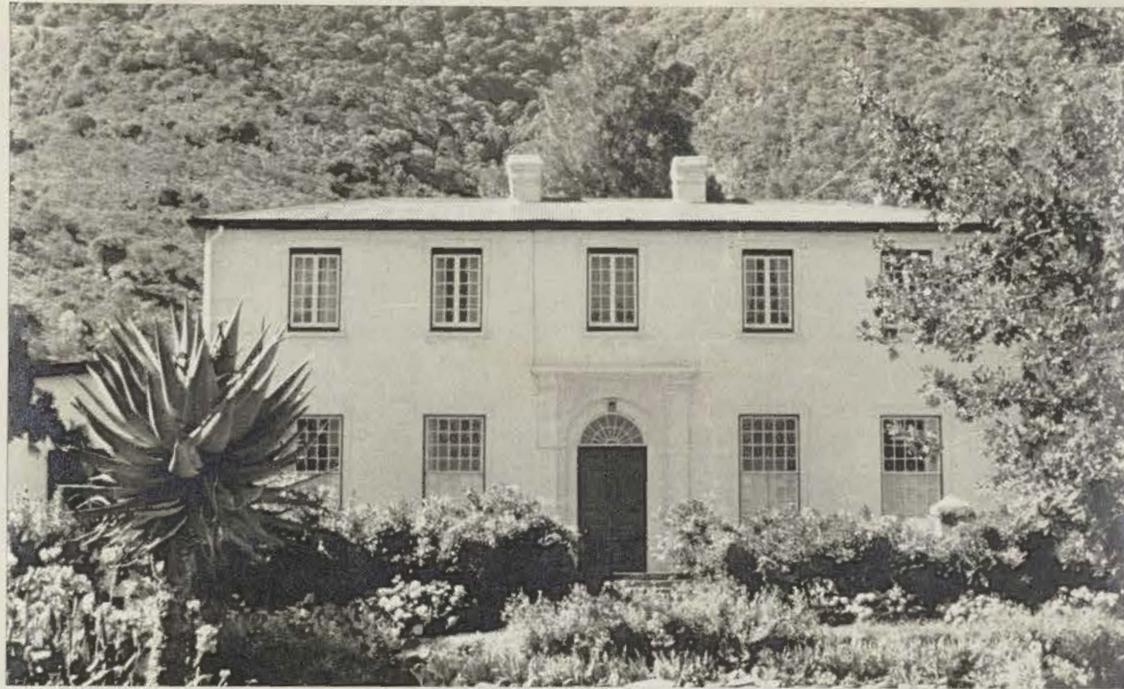
124. Somerset East Drosty, facade.
