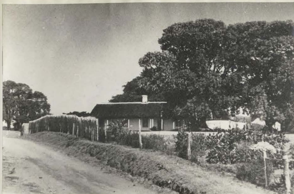
28. 'Greenfountains', distant photograph. The thatched roof survives under later galvanized iron. The photograph has been retouched to show the original appearance.
