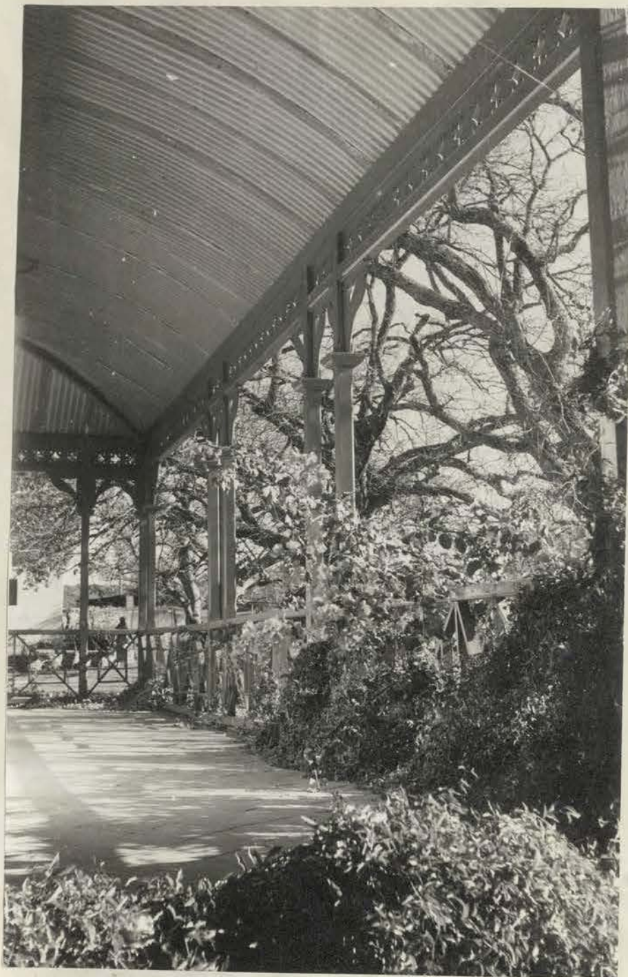
64. 'Oatlands', Grahamstown. Interior of the (mid-Victorian) veranda.
