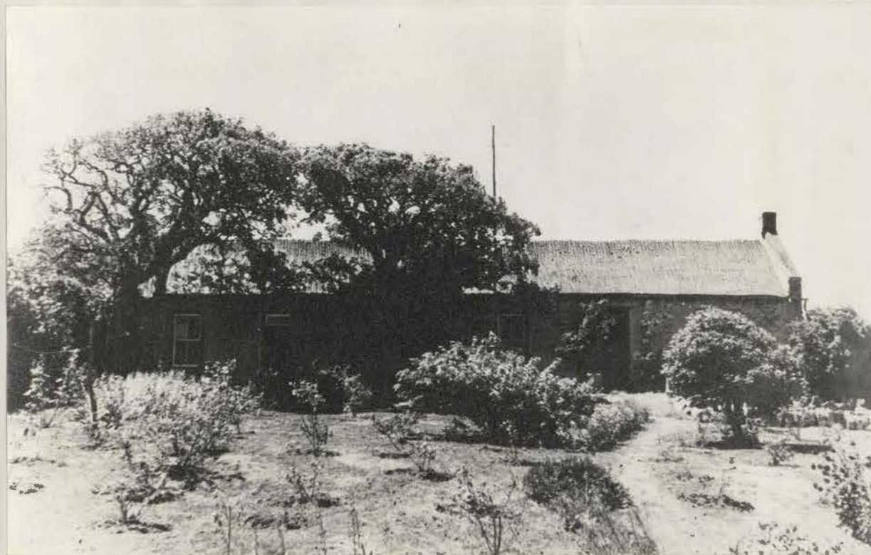
43.B, 44. 'Tharfield', Kleinemonde. South facade and plan. (The later additions are shown shaded).
