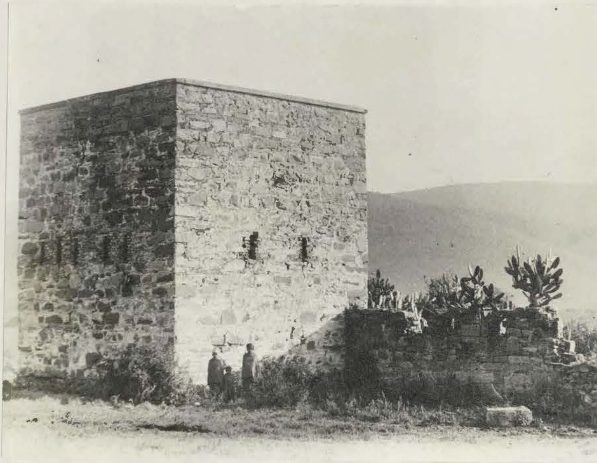
106. Tower of Double Drift Fort.
