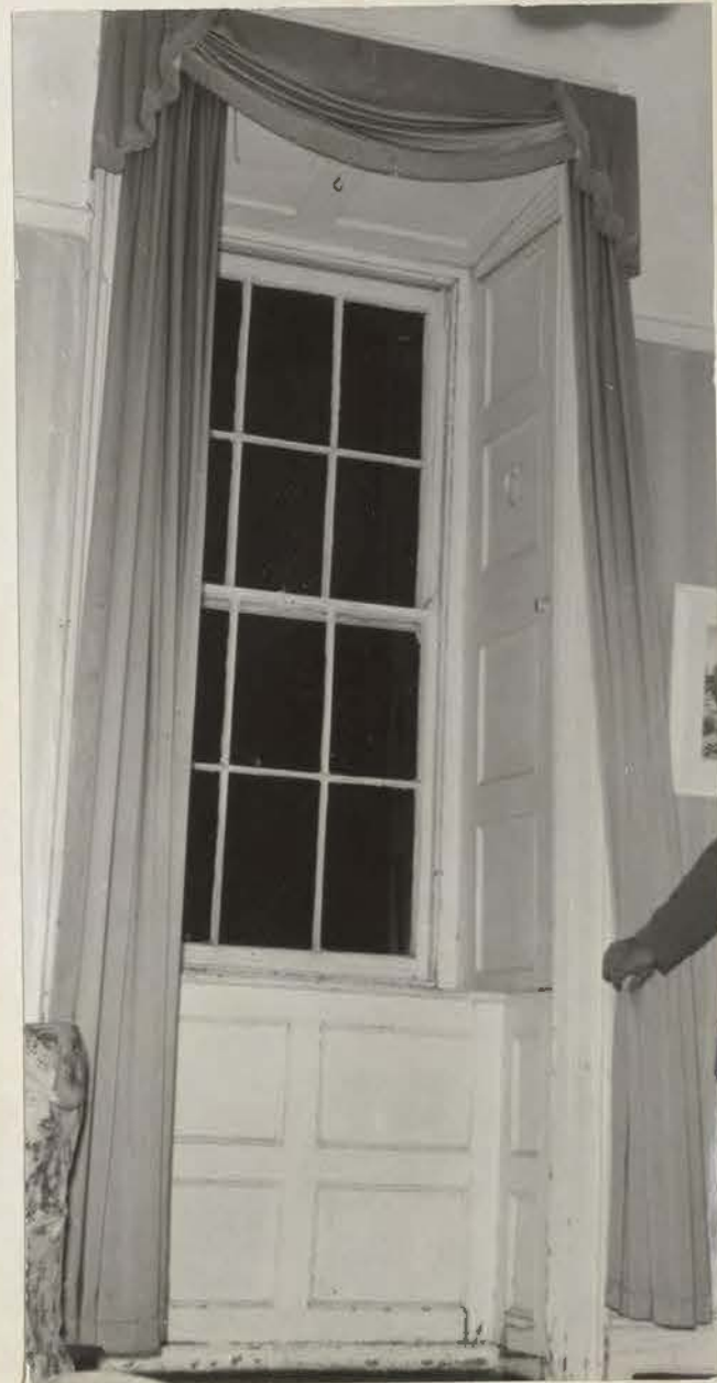
146. Window in a house on the corner of High and Somerset Streets, Grahamstown, which at one time served as the Lieut.-Governors Offices.
