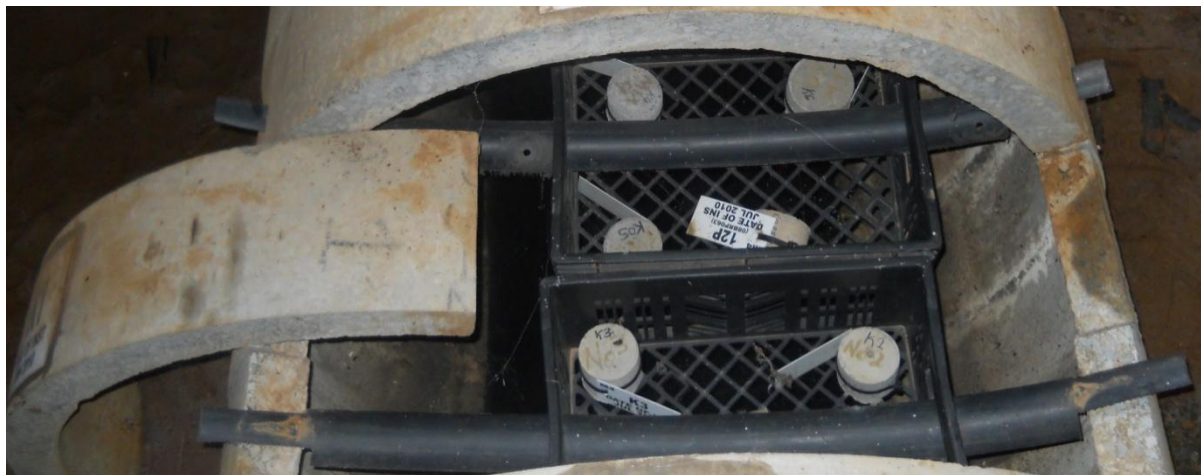
Figure 5.6 The experimental setup showing installation of cylindrical samples in Virginia experimental sewer.
