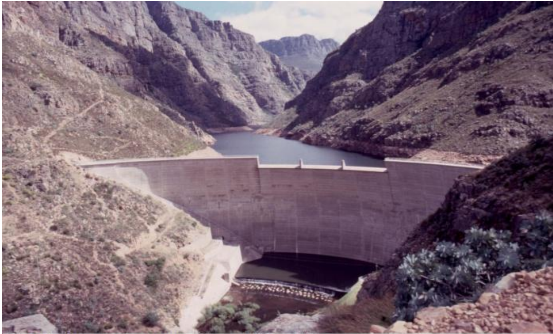
Figure 21: Roode Elsberg Dam located in Worcester Western Cape, South Africa
