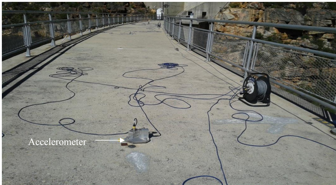
Figure 29 : Field testing of Roode Elsberg dam based method that identifies the operational modal parameters of the dam.
