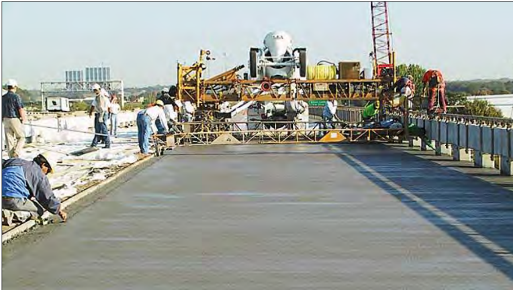
Figure 2-1: Concrete overlay used to repair a bridge deck ( http://www.wildcatcompanies.com/concrete.html )
