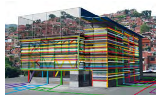
Figure 7.22: Vertical Gymnasiums in Caracas, Venezuela (Source: UN-Habitat, 2016)
