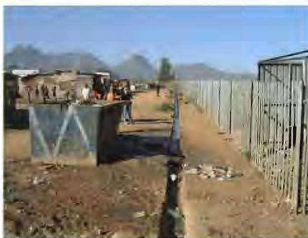
Figure B1.6: Stormwater channel at Fairyland (Winter, 2006)
