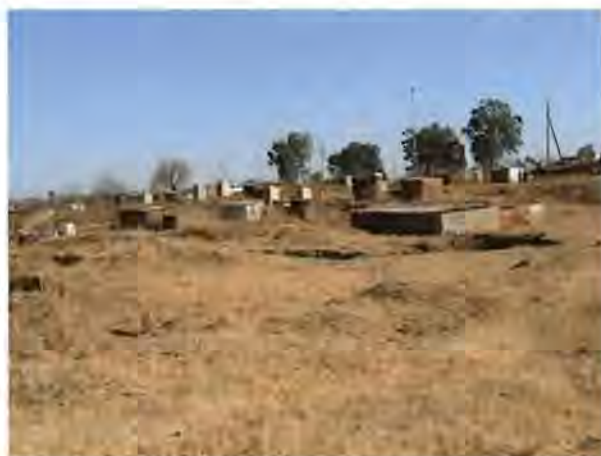
Figure D3.2: Shacks situated on moderate slopes on banks of Mzintlava River (Winter, 2006)
