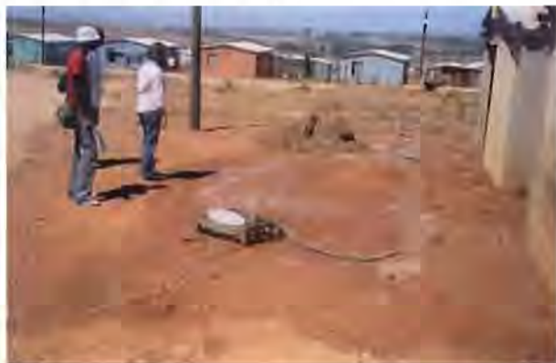
Figure B1.13: Water supply at Lingelethu (Armitage, 2006)
