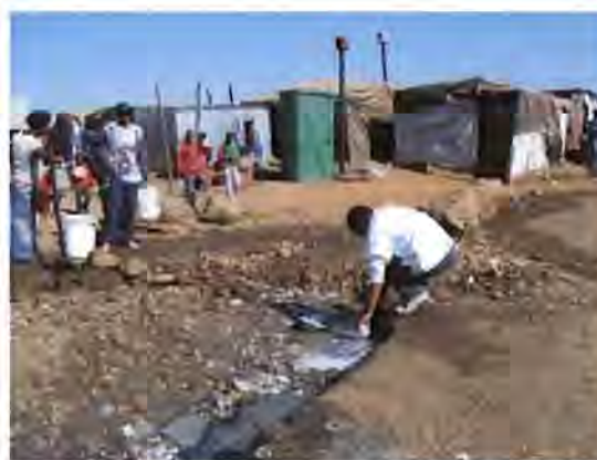
Figure B6.4: Stormwater drain at Freedom Square (Sichone, 2006)
