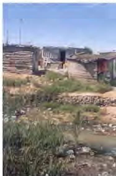
Figure B1.12: Stormwater channel, Khayelitsha (Sichone, 2006)
