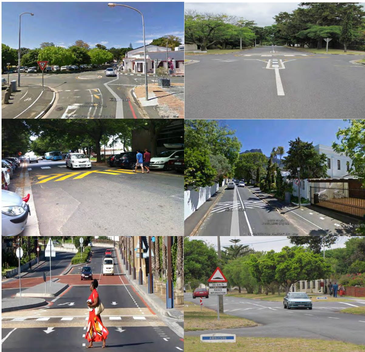
Figure 52: Sample photos of selected traffic calming measures
