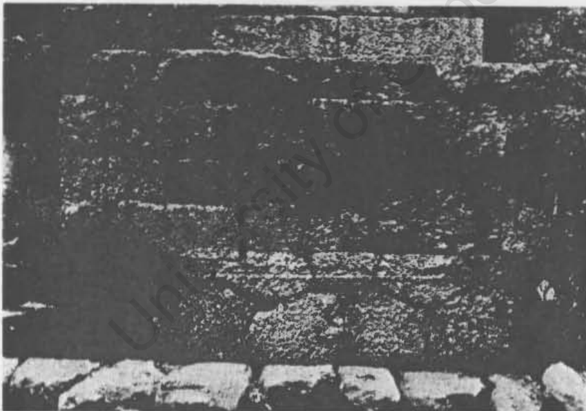
224 Section of the Themistoklean Wall near the Sacred Gate. The lower part of the wall, 0.75 m. high, is of Acropolis limestone, the upper part of poros.
