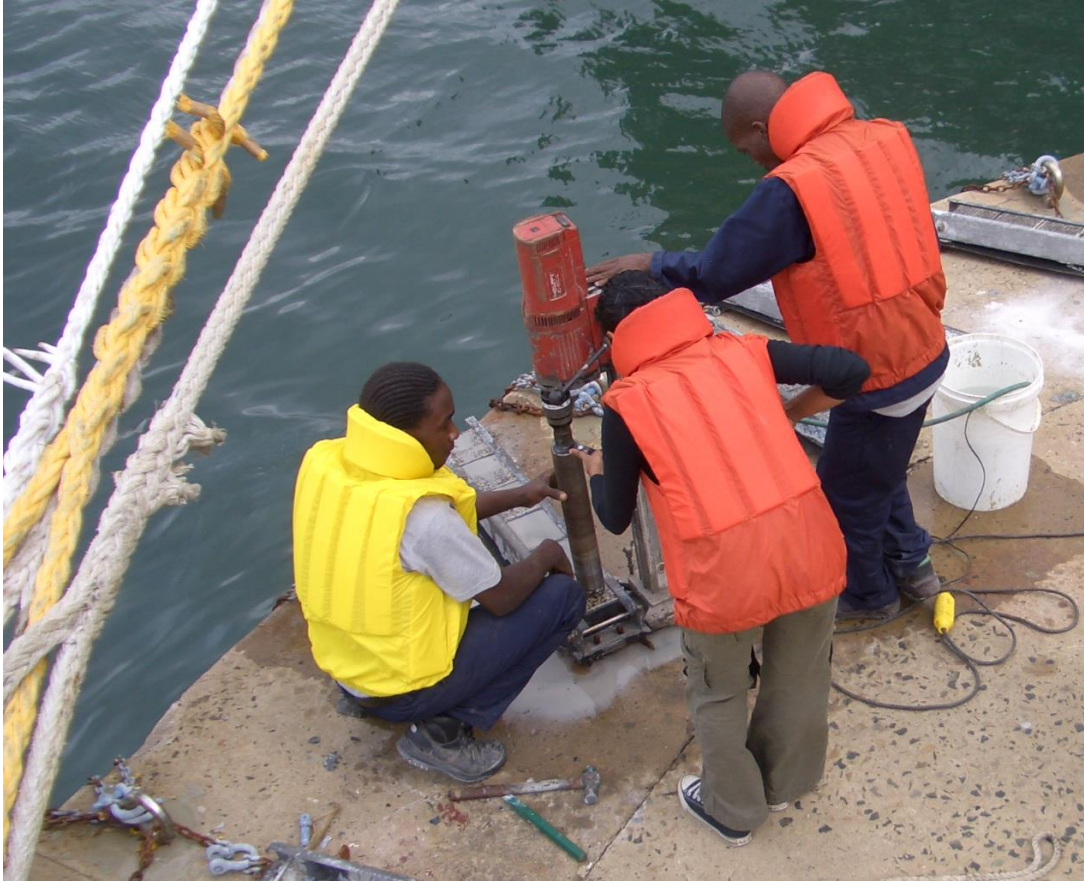
Figure 3.9: Removing of core samples on site (Durban)
