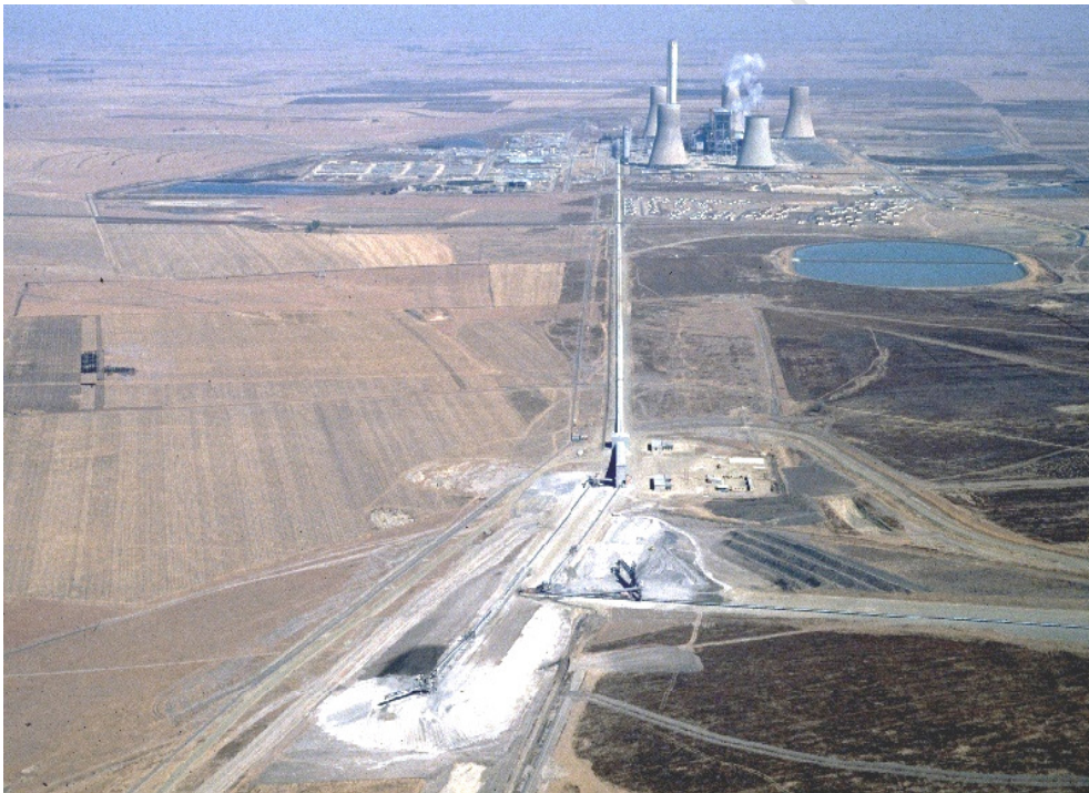
Figure 2: Aerial image depicting overland ash conveyors which culminate in ash dumps (foreground), and cooling towers of wet cooling system shown adjacent of the power station (background)
